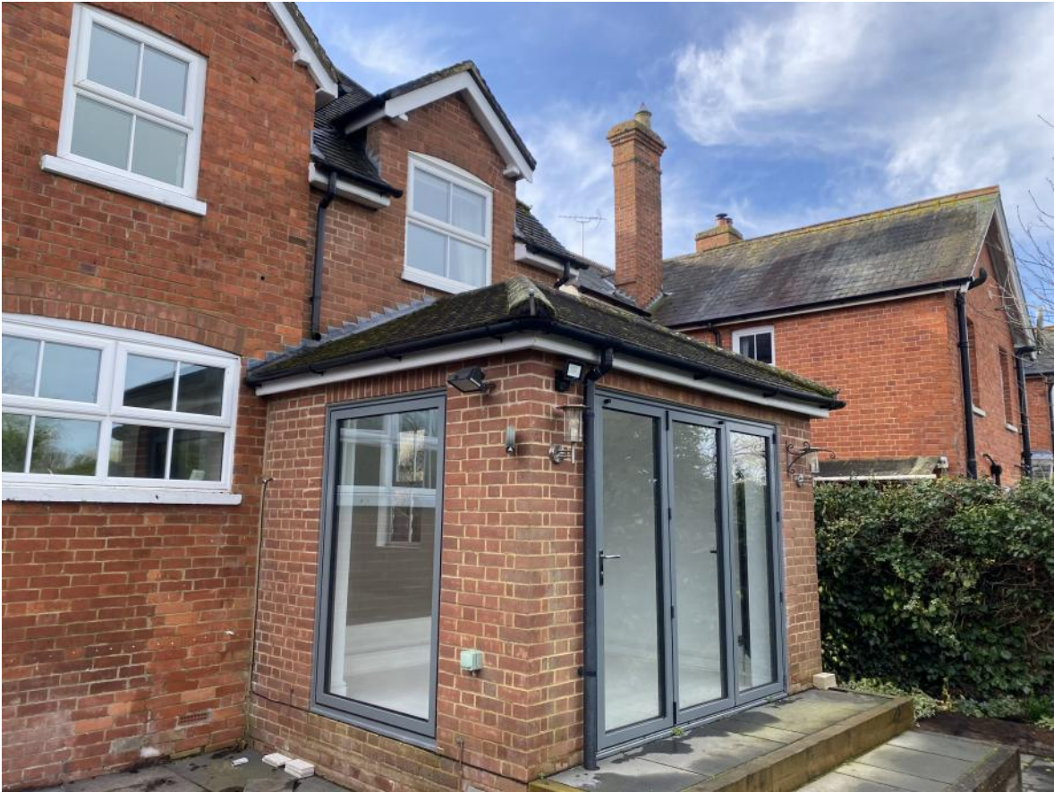
View showing single storey extension to be demolished
