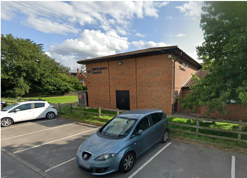
Figure 1 – photograph showing the site as existing
