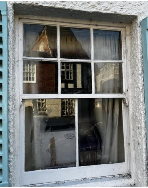
Existing timber sash windows
