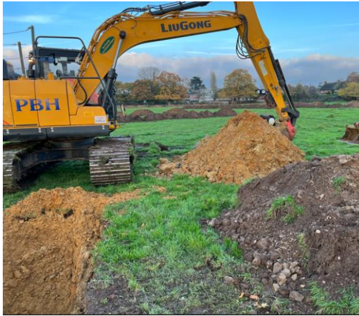
Figure 2.5: Archaeological excavations and residences near site.
