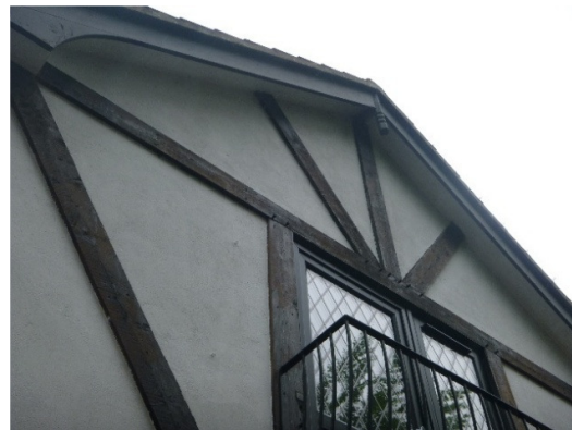
Photograph 7. Render tight on the front gable end.
