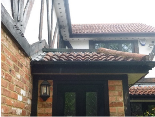
Photograph 8. Lead flashing tight at the join of the porch with the main house.
