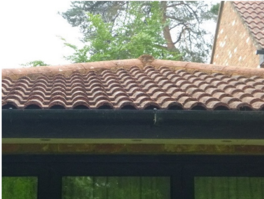
Photograph 5. Hip tiles fully mortared on the rear single storey roof extension.
