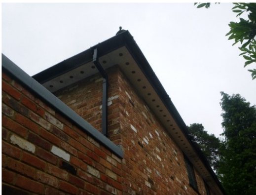
Photograph 6. Soffit boxes tight to the brick work walls (rear elevation).
