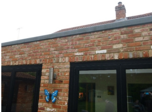
Photograph 10. Flat roof extension with a tightly fitted roof.
