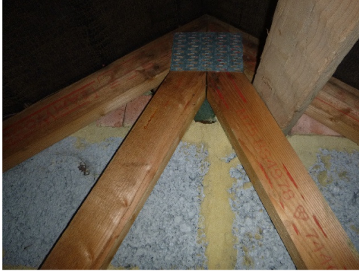
Photograph 17. Tight block work at the gable end.
