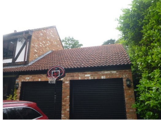
Photograph 4. Tight interlocking tiles on the roof of the garage.
