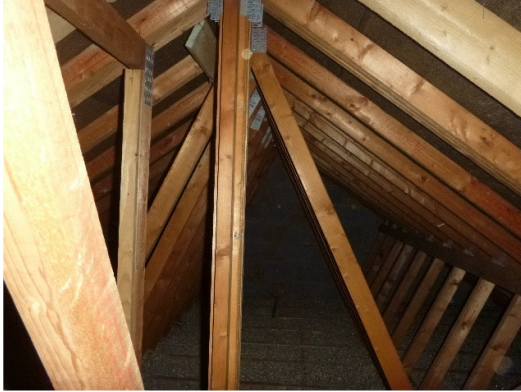
Photograph 11. Roof space of trussed rafter construction.
