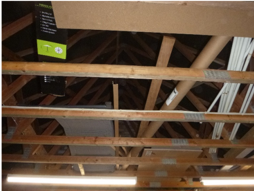
Photograph 19. Internal view of the garage.
