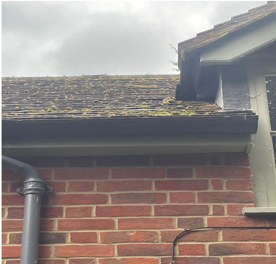
Plate 14: An image showing loose tiles on the roof and gaps in the soffit
