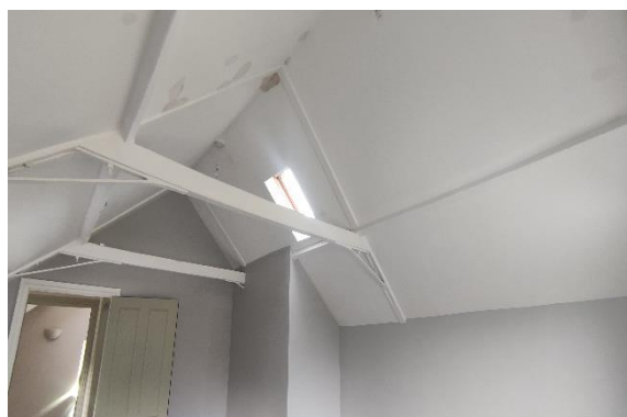
Photograph 10. Room within the roof of the coach house.
