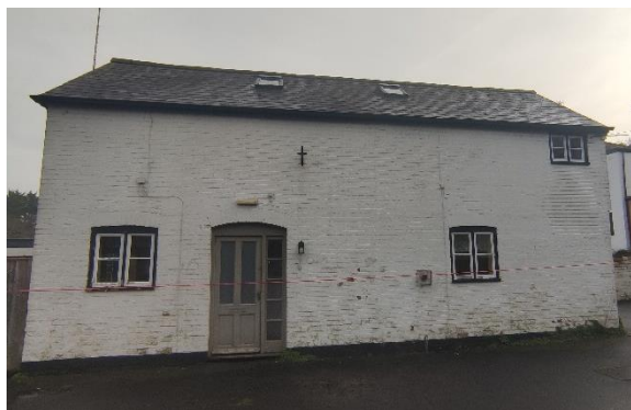
Photograph 7. Western elevation of the coach house.
