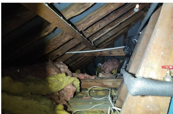
Photograph 5. Area of loft void above eastern section of roof. Obstructed by water tank.
