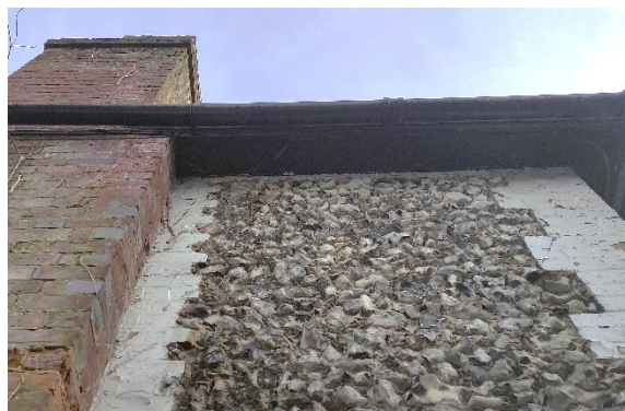
Photograph 4. Example of tight-fitting boxed eaves.
