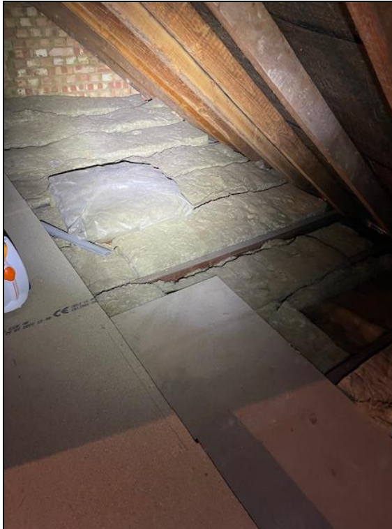
Photograph 5: Main house loft space.
