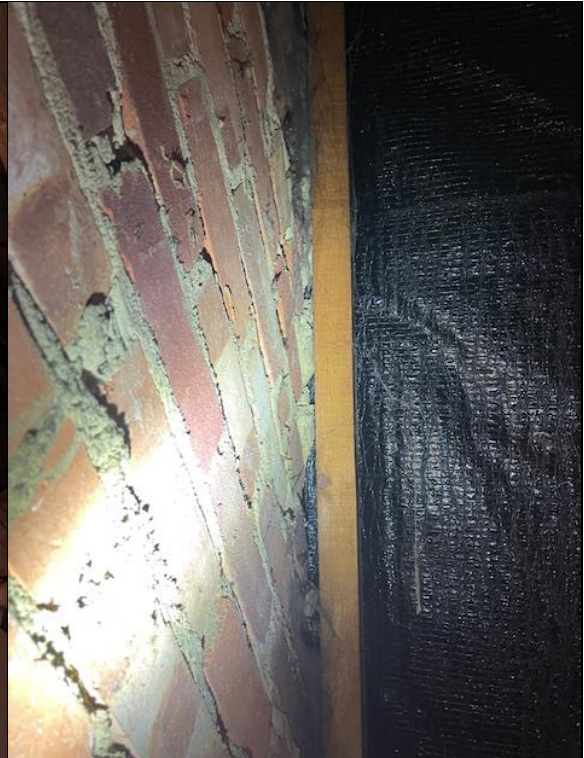
Photograph 6: Main house loft space.
