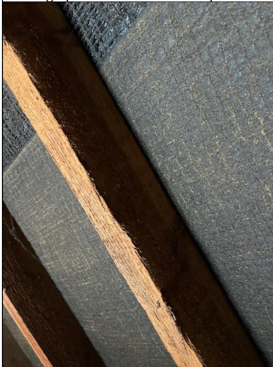
Photograph 3: Main house loft space.
