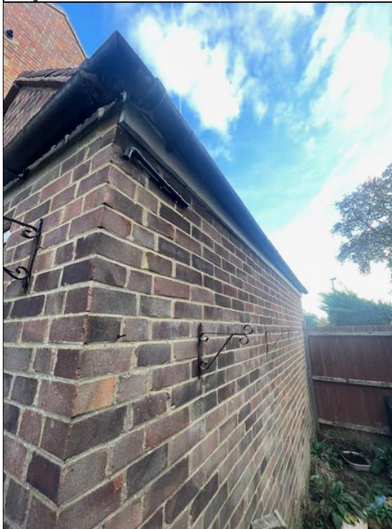
Photograph 15: Adjacent brick-built garage.
