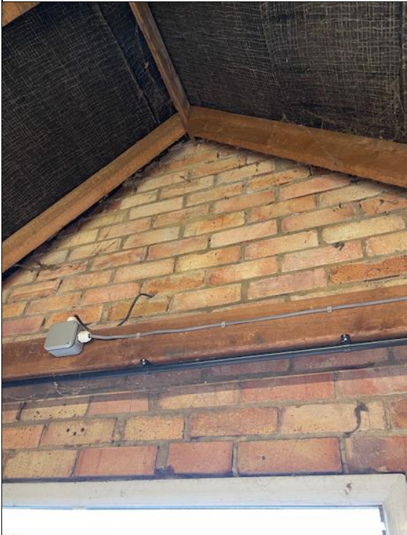
Photograph 19: Garage interior and loft area.
