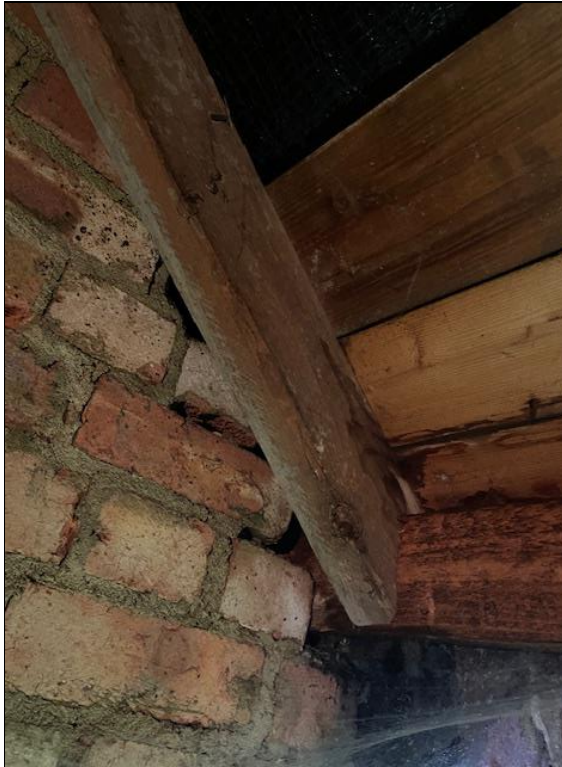
Photograph 9: Main house loft space.
