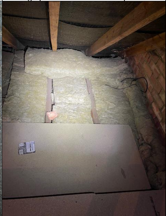
Photograph 4: Main house loft space.
