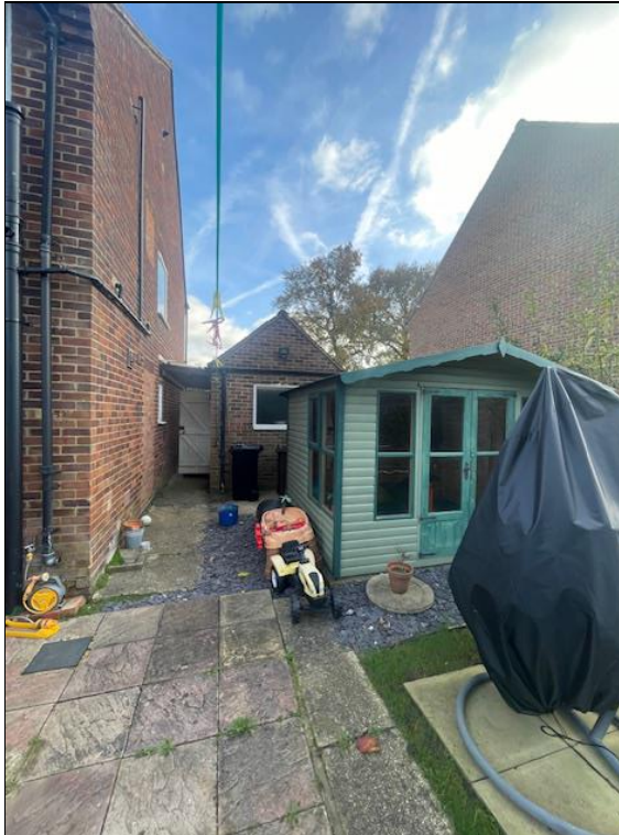
Photograph 13: Side elevation patio with adjacent wooden shed.
