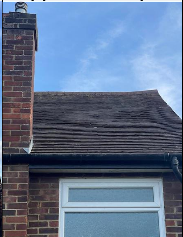
Photograph 12: Roof tiles in good condition with no lifts.
