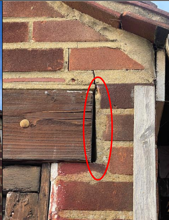
Photograph 22: Gap between the wood and the mortar - could be fully inspected.
