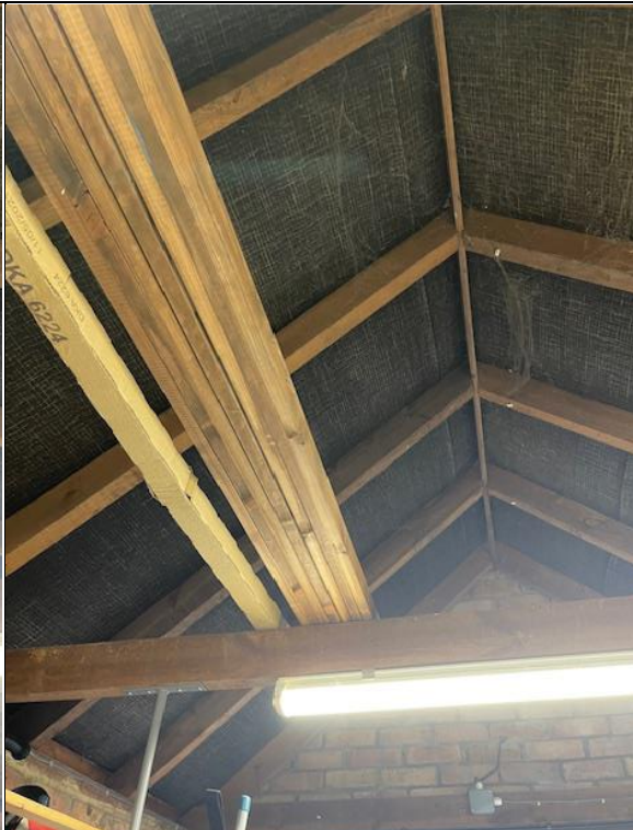
Photograph 18: Garage interior and loft area.
