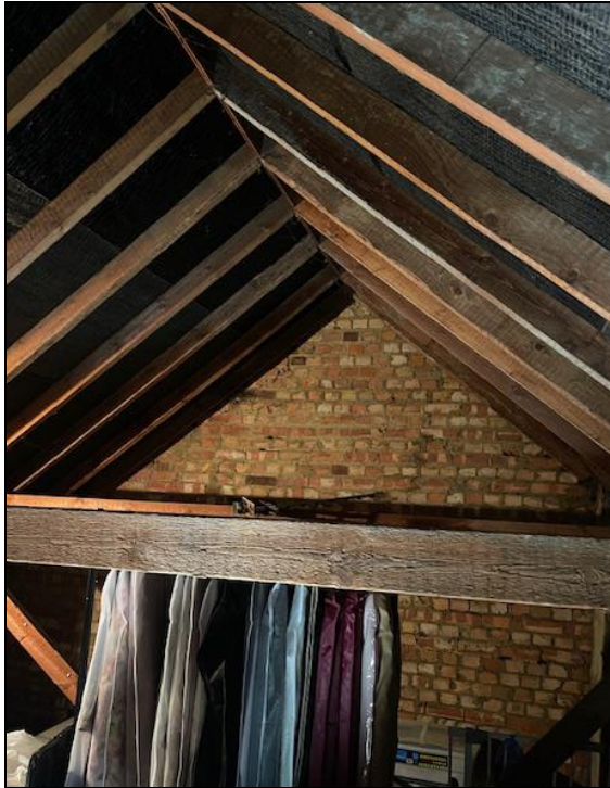
Photograph 1: Main house loft space.
