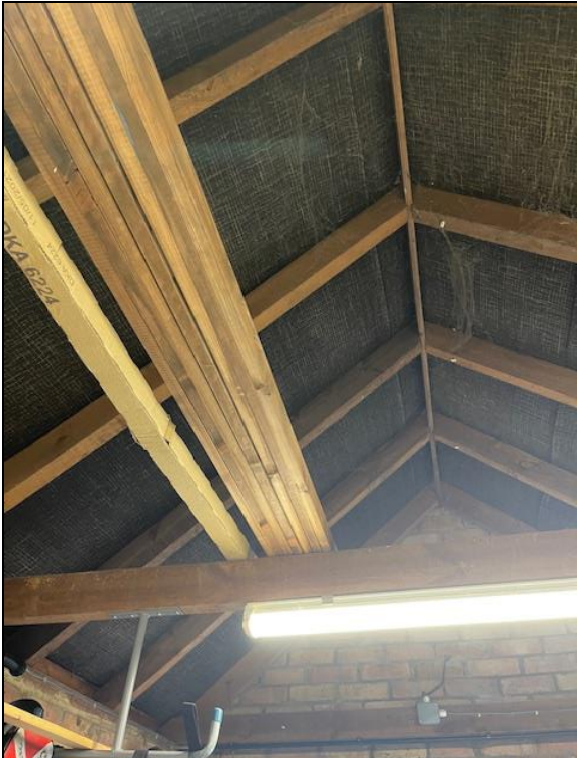
Photograph 17: Garage interior and loft area.
