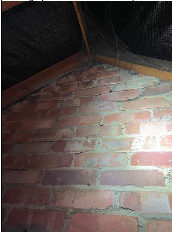
Photograph 7: Main house loft space.
