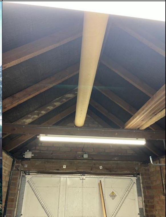
Photograph 16: Garage interior and loft area.
