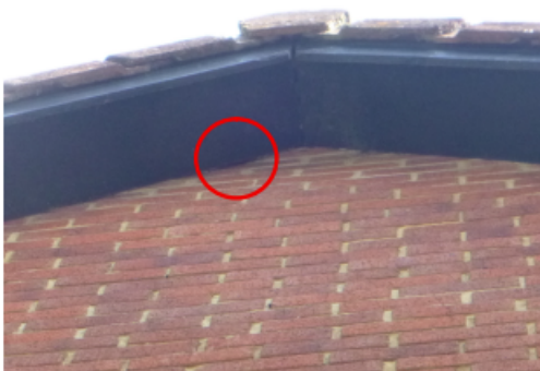
Photograph 7. Gap under soffit near apex of the gable (southern elevation).
