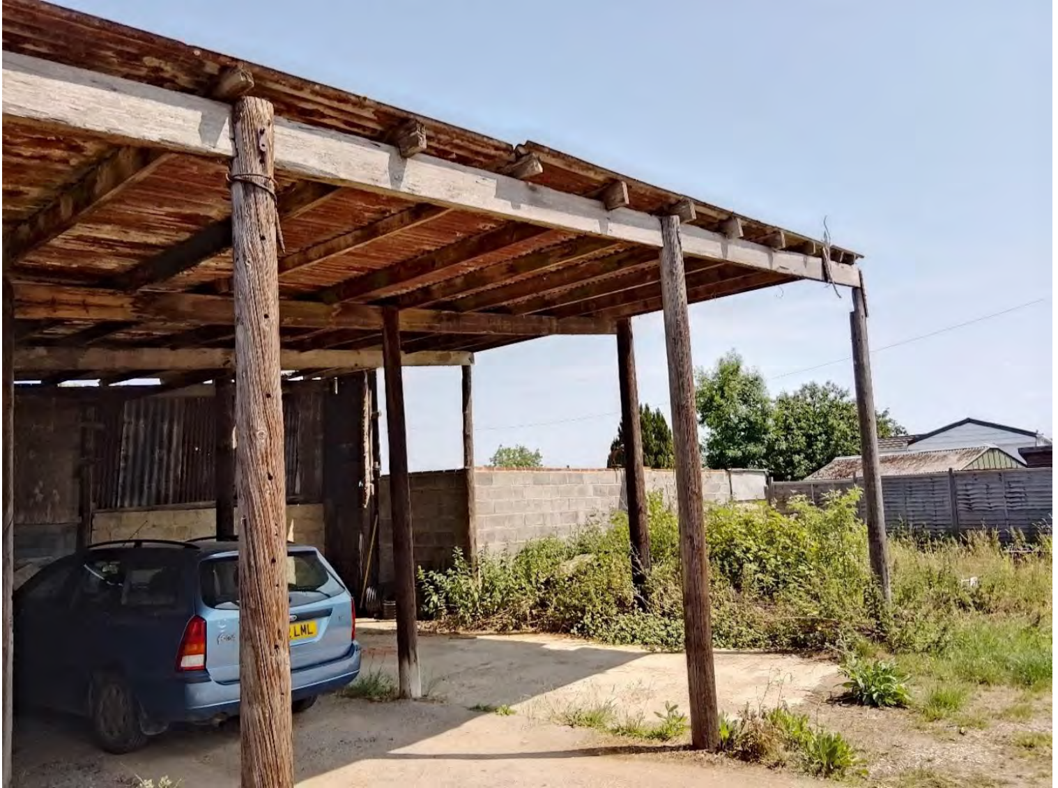
View of a covered structure in the west of the site with possible asbestos roofing material present looking northeast. The visible concrete block wall and wooden fencing form the northern boundary in this section of the site. Surface covering is poured concrete/concrete slabs and compacted gravel with overgrown vegetation.
