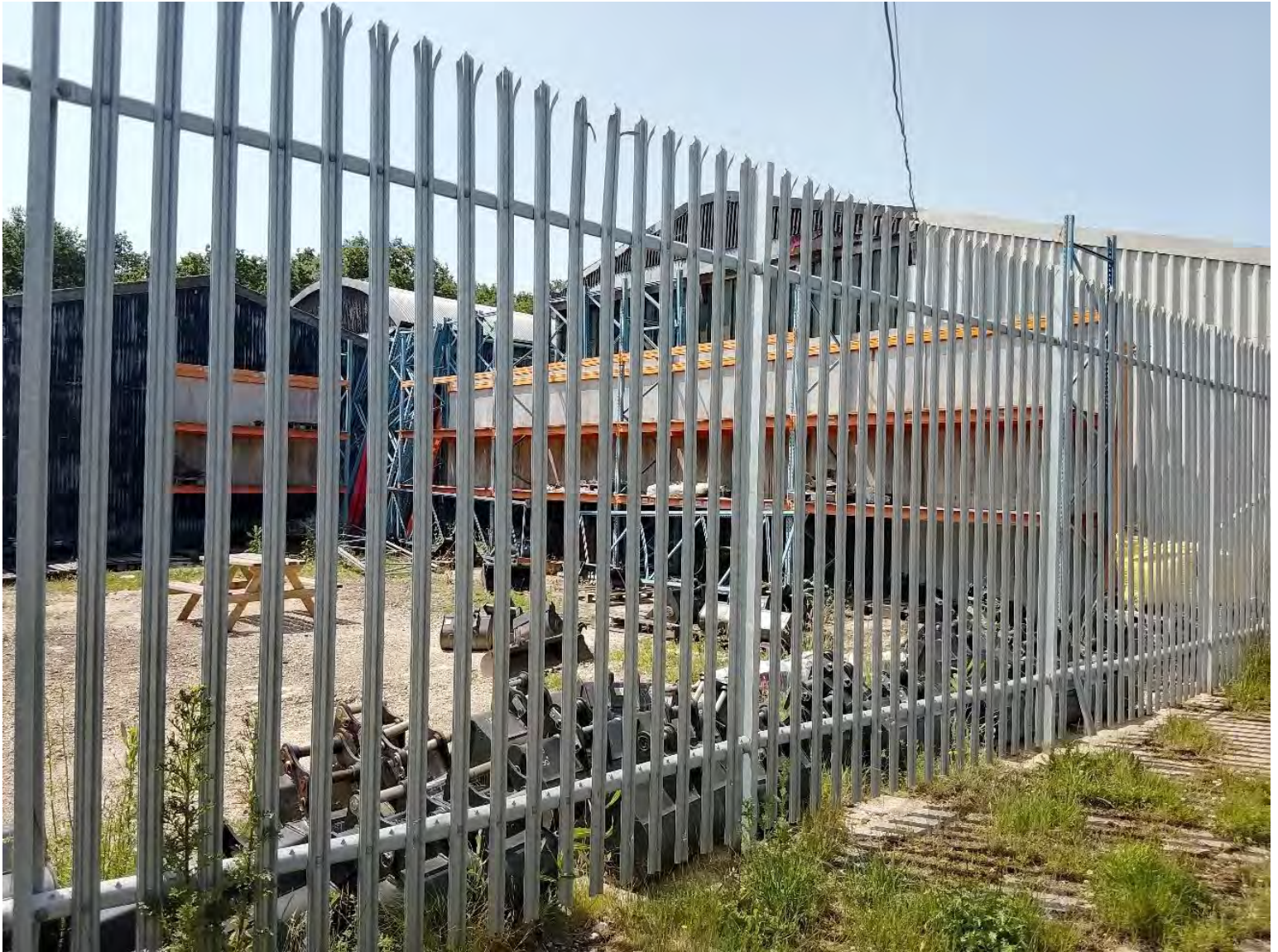
View of metal palisade fencing with an external storage area beyond in the west of the site looking southwest. Surface covering is poured concrete/concrete slabs and compacted gravel with overgrown vegetation.
