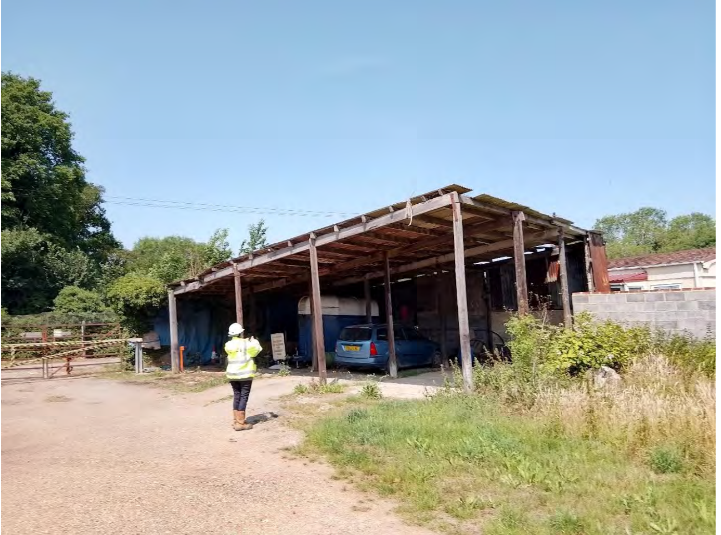
View of a covered structure in the west of the site with possible asbestos roofing material present looking northwest. The vehicular access gate off Whitehouse Farm (road) is visible on the left of the image. Surface covering is poured concrete/concrete slabs and compacted gravel with overgrown vegetation.
