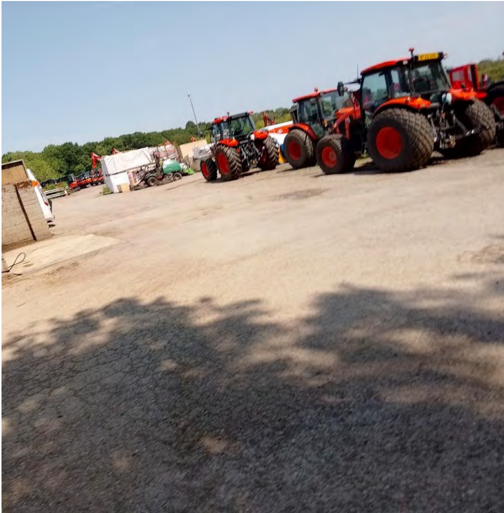
View of the southern vehicle and machinery storage yard in the centre of the site looking north. Surface covering is poured concrete, cracking is visible.
