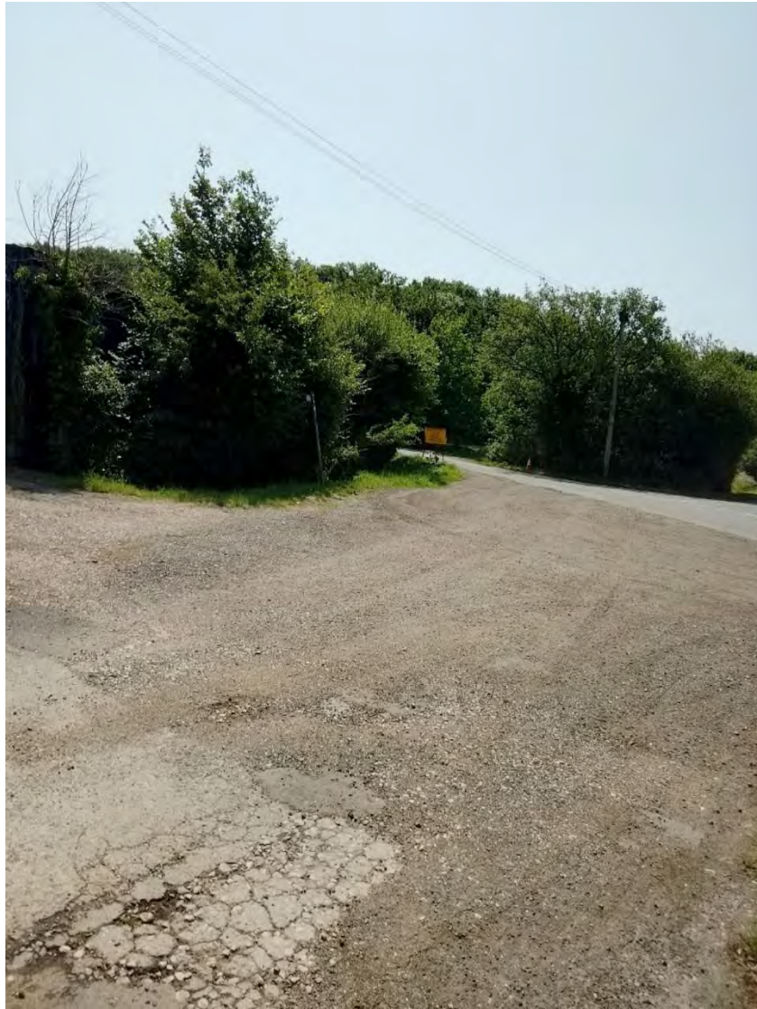
View of the road access at the junction of Yew Tree Lane and White House Lane looking south. Surface covering is compacted gravel and concrete slabs.
