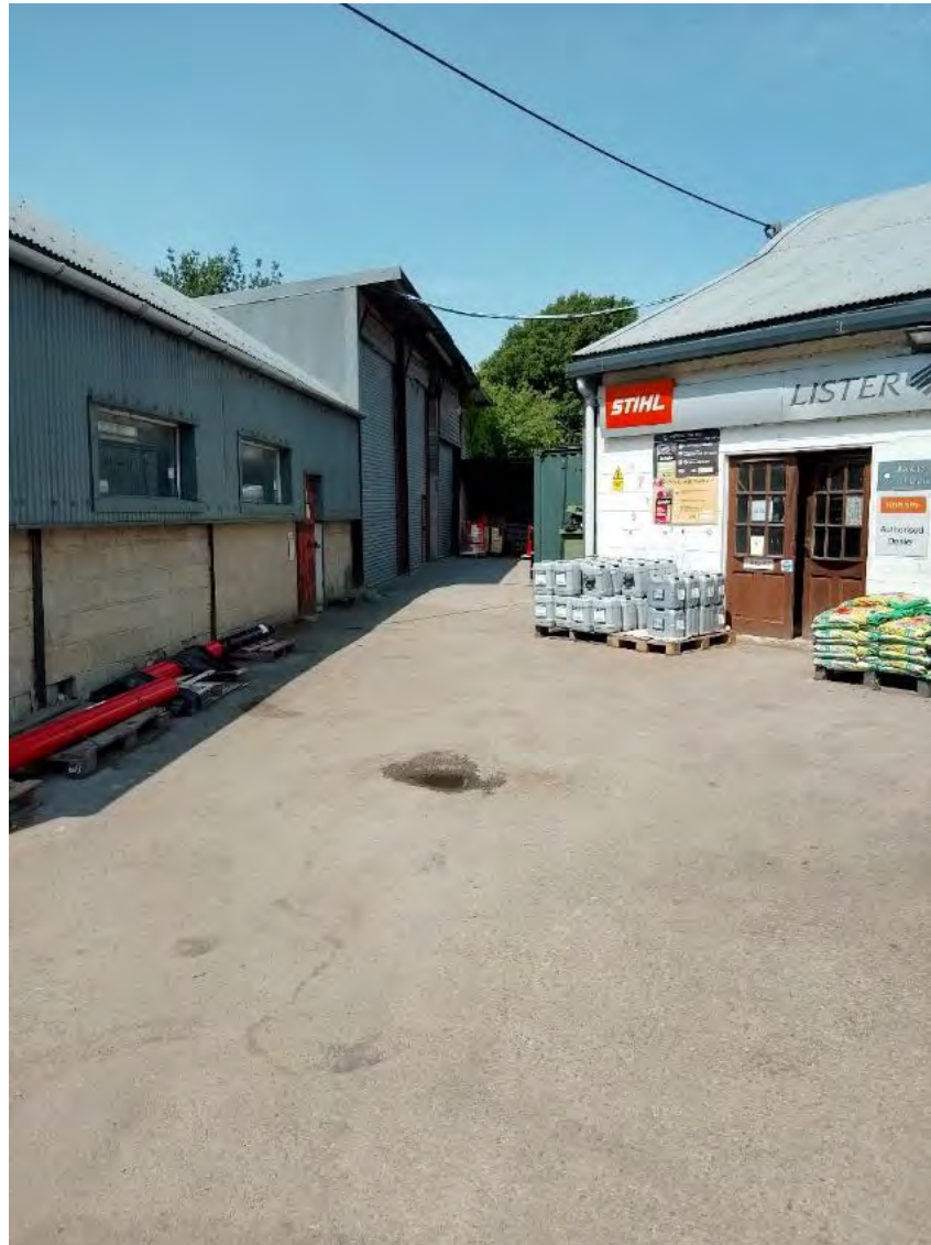
View of the retailer's yard looking northwest. Further corrugated metal and concrete block structures of unknown purpose are visible in the far distance. Overhead cables are visible crossing the site. Surface covering is poured concrete.
