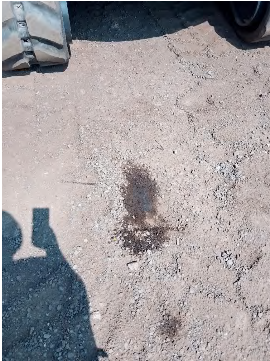
Photograph of minor surface staining caused by an unknown substance in northern vehicle and machinery storage compound in the centre of the site. Surface covering is compacted gravel.
