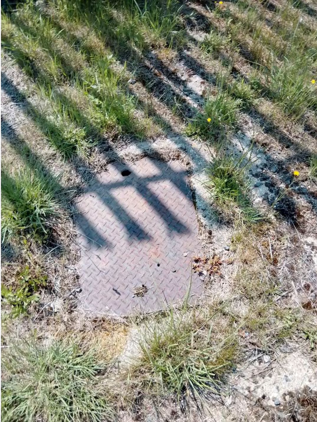
Photograph of a cover, below which is a possible underground structure or tank.
