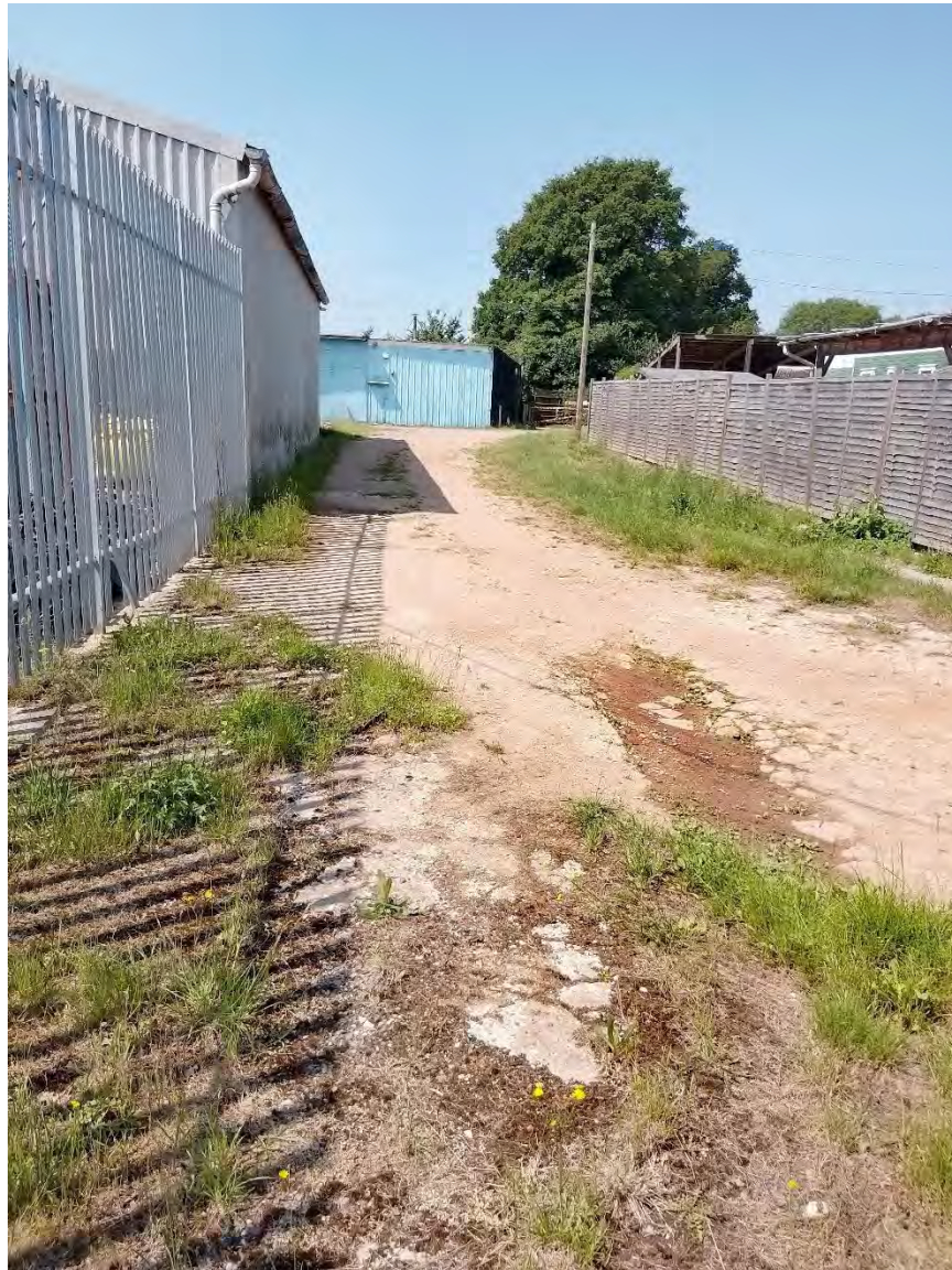
View of vehicular access road running east/west through the west of the site looking west. The wooden fence on the right of the image forms the northern boundary in this part of the site. Surface covering is poured concrete/concrete slabs and compacted gravel with overgrown vegetation.
