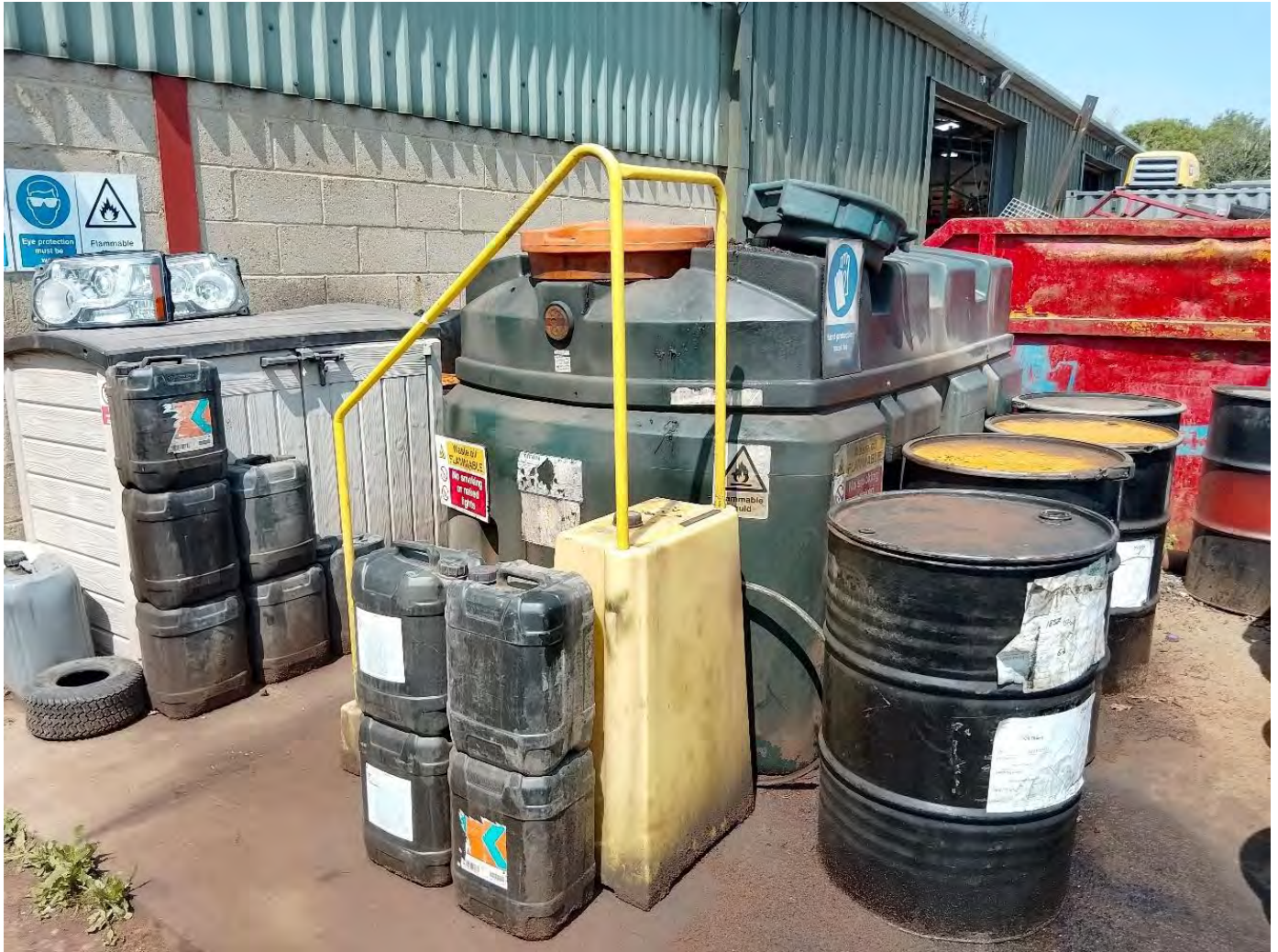
Photograph of oil storage facilities sited on a concrete slab with visible staining and discoloration in the center of the site. Concrete brick and corrugated metal vehicle maintenance workshops are visible in the background.
