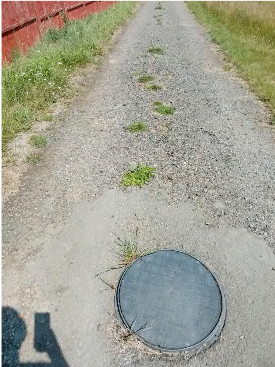
Photograph of field access road surface and integrated manhole in the west of the site running north/south. Surface covering compacted and loose gravel with scattered vegetation.
