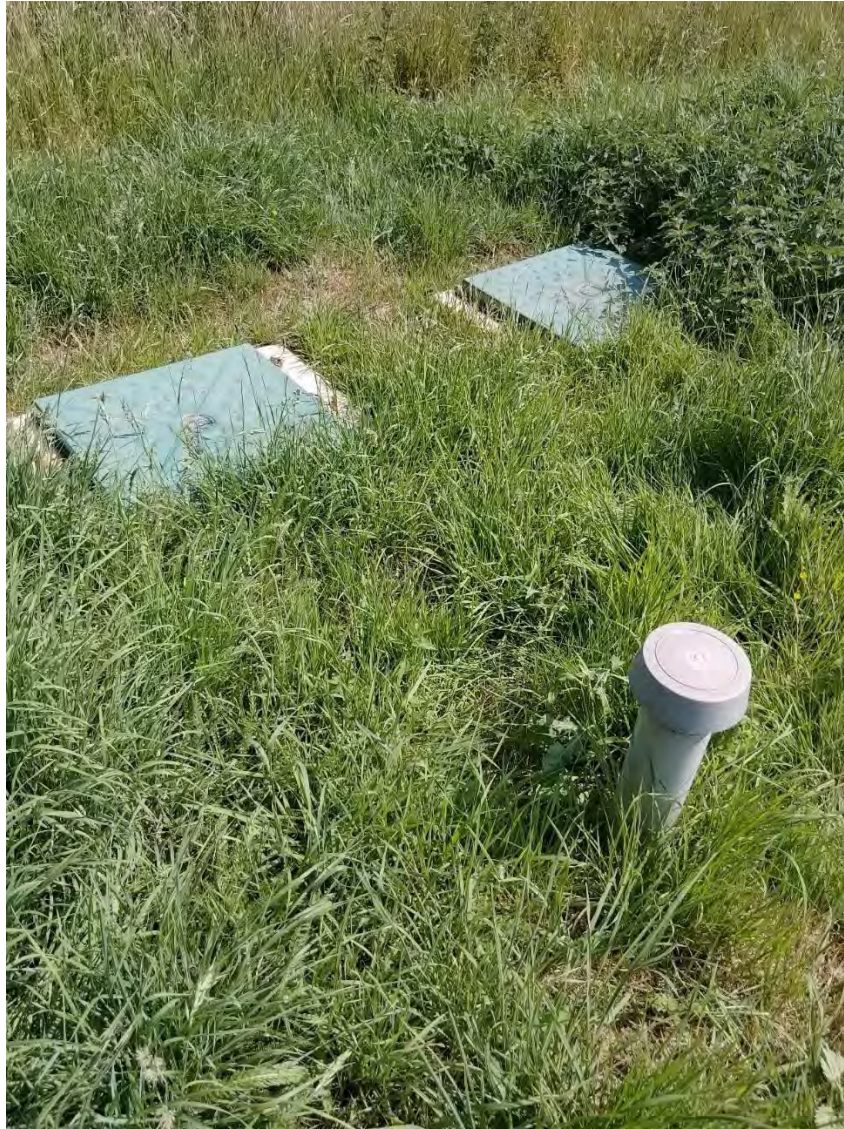
Photograph of septic tank inspection and ventilation covers in the field beyond the northern boundary of the site.
