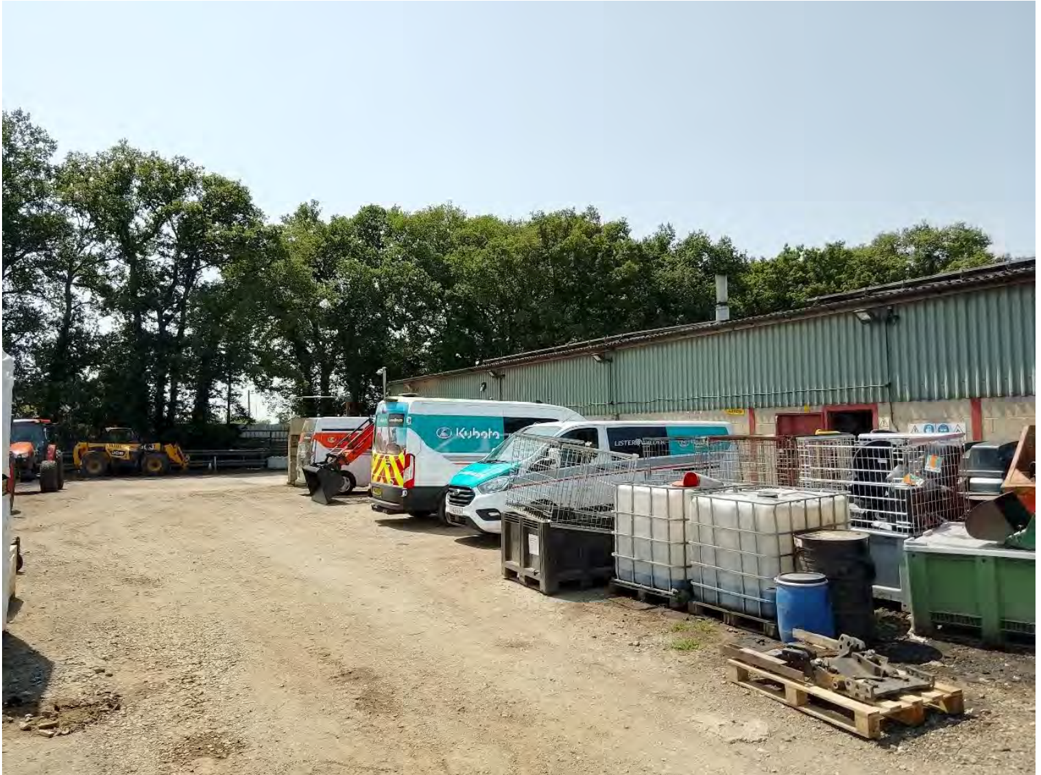
View of concrete block and corrugated metal vehicle maintenance workshops in the centre of the site looking south. Surface covering is compacted gravel and poured concrete.
