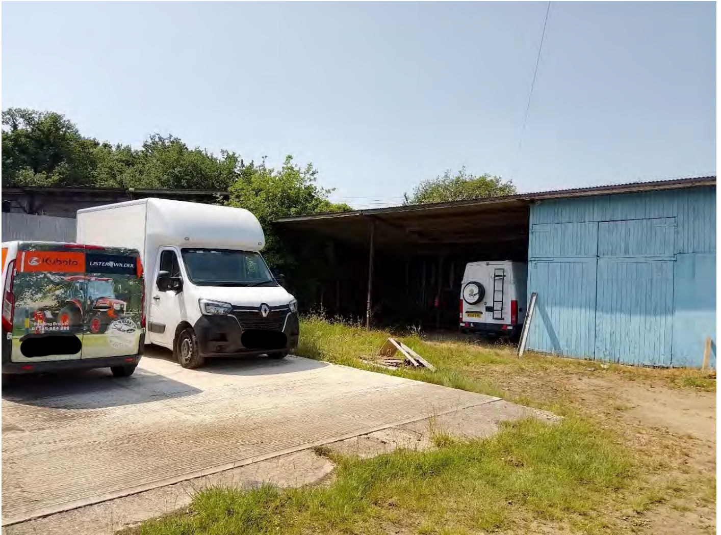
View of a corrugated metal and wooden structure, including a covered vehicle bay and parking area in the west of the site looking southwest. Surface covering is poured concrete/concrete slabs and compacted gravel with overgrown vegetation. Photo 19 was taken in the space between the parking area and the covered vehicle bay.
