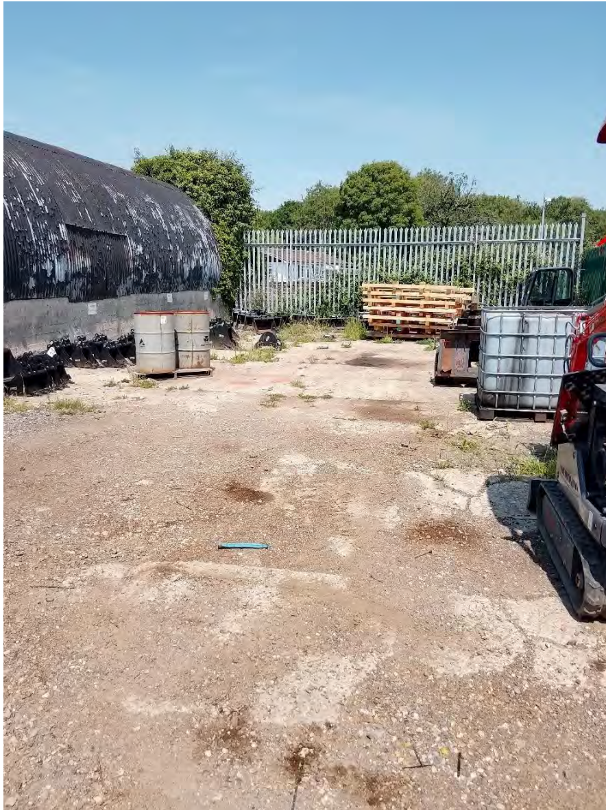
View of external storage area in the western area of the site looking north. Also visible is a concrete block and corrugated metal structure and vehicle oil IBCs. Surface covering is poured concrete and concrete slabs.
