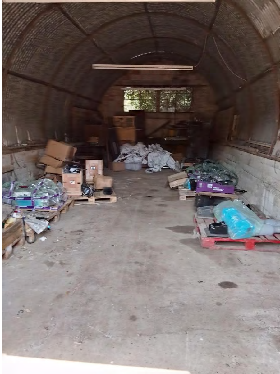
Internal view of concrete block and corrugated metal structure with concrete slab flooring in the western area of the site looking north.
