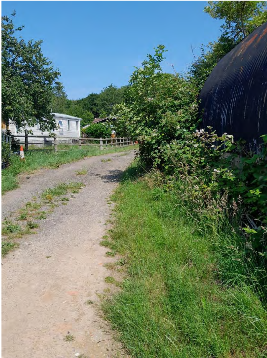
View of the existing field access running north/south outside of the site boundary looking north. Surface covering is poured concrete/concrete slabs and compacted gravel with overgrown vegetation.
