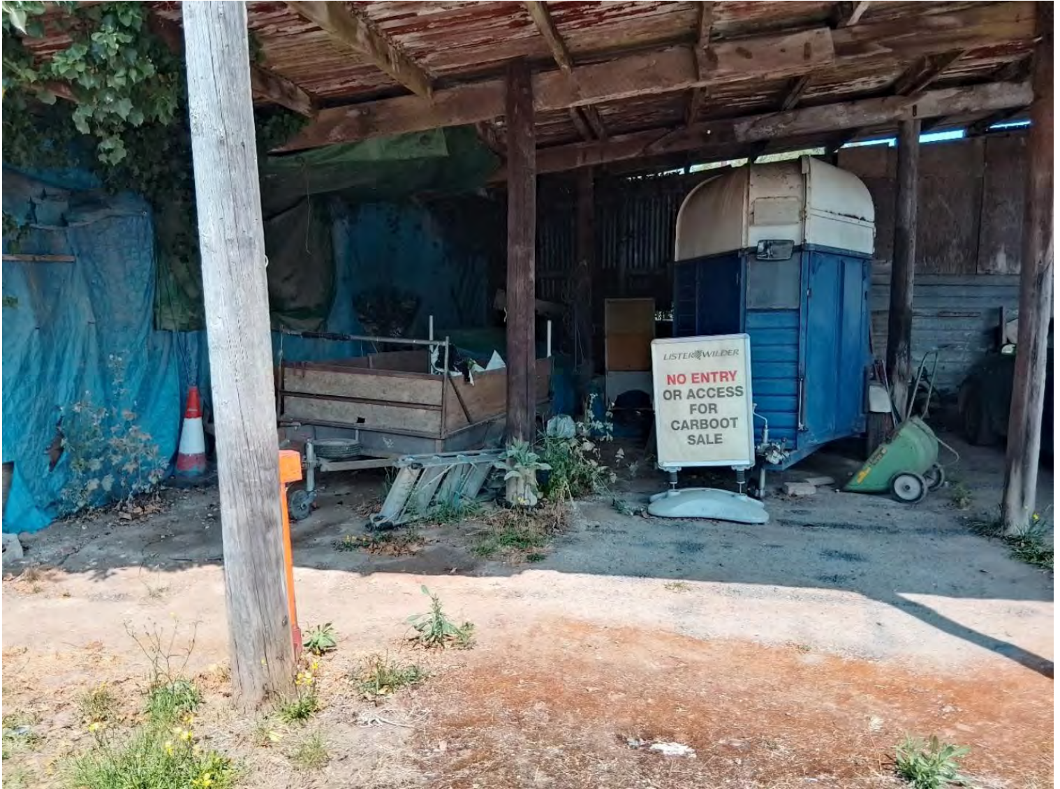
View of various items stored under a covered structure with possible asbestos roofing material present in the west of the site looking north. Surface covering is poured concrete/concrete slabs and compacted gravel with overgrown vegetation.
