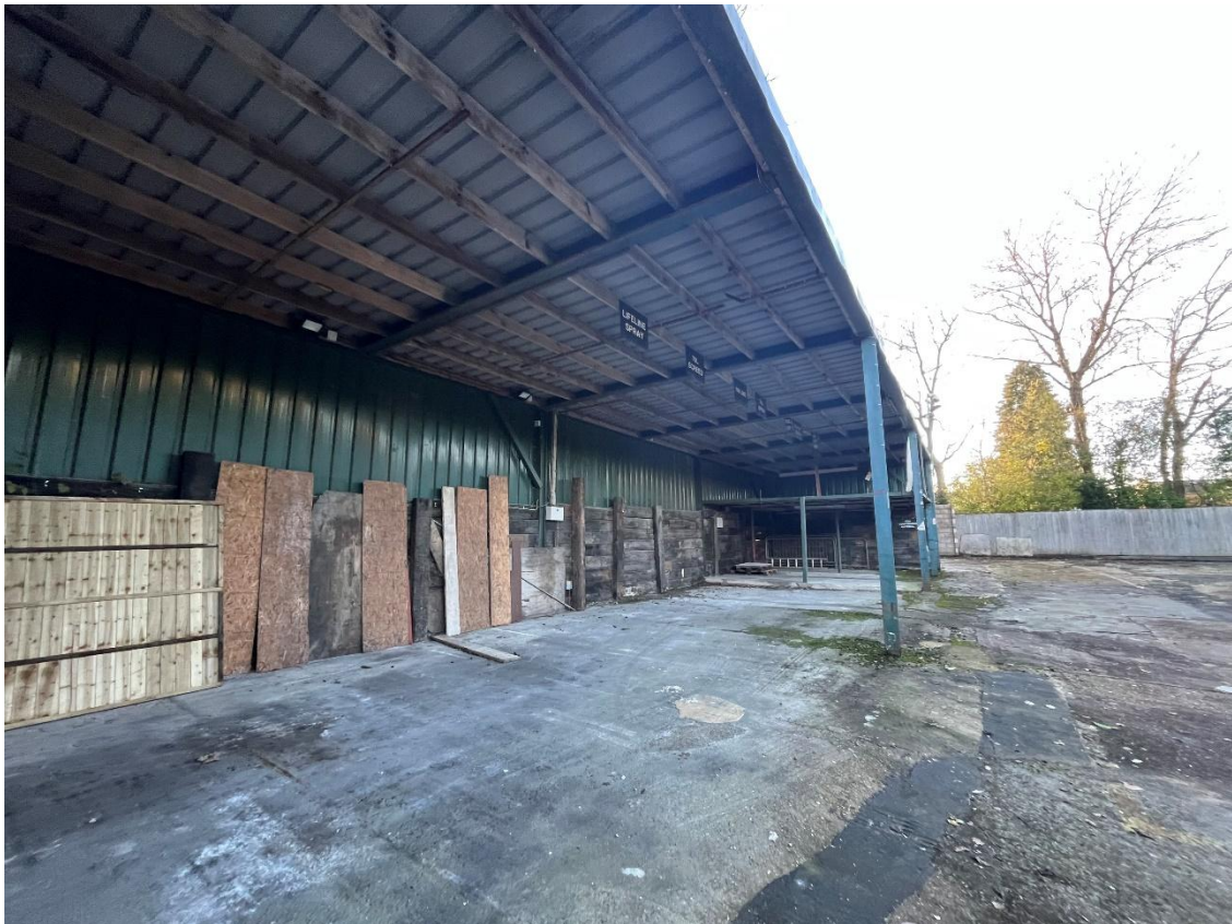
Figure 6. Block B open bays looking west.
