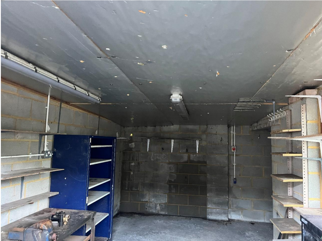
Figure 7. Interior of block B workshop looking south.
