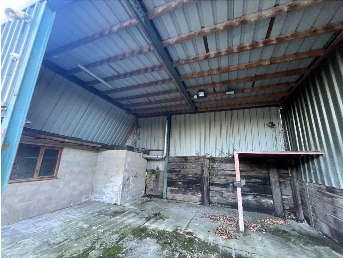
Figure 5. Block B easternmost open bay and workshop looking south.
