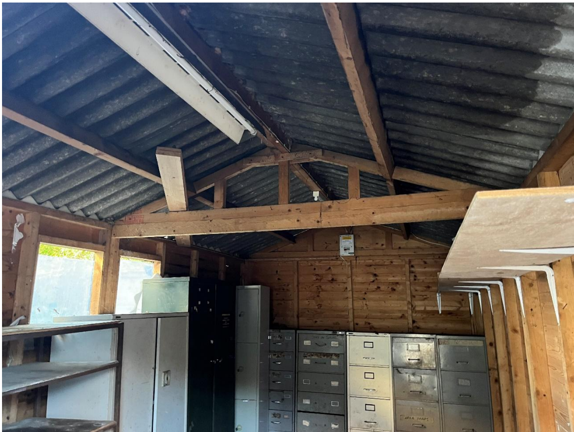
Figure 9. Block C interior looking east.
