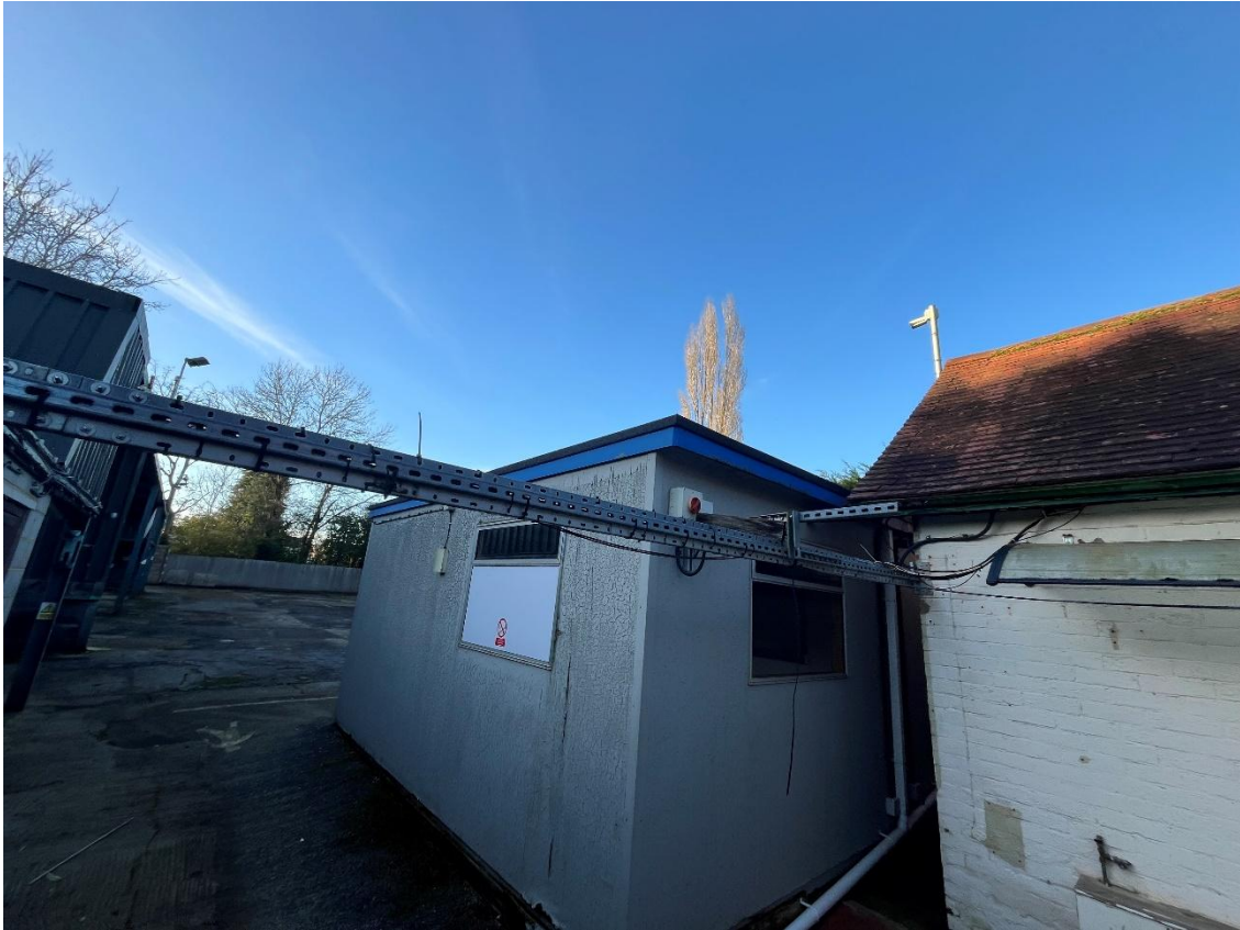
Figure 4. Block A looking west
