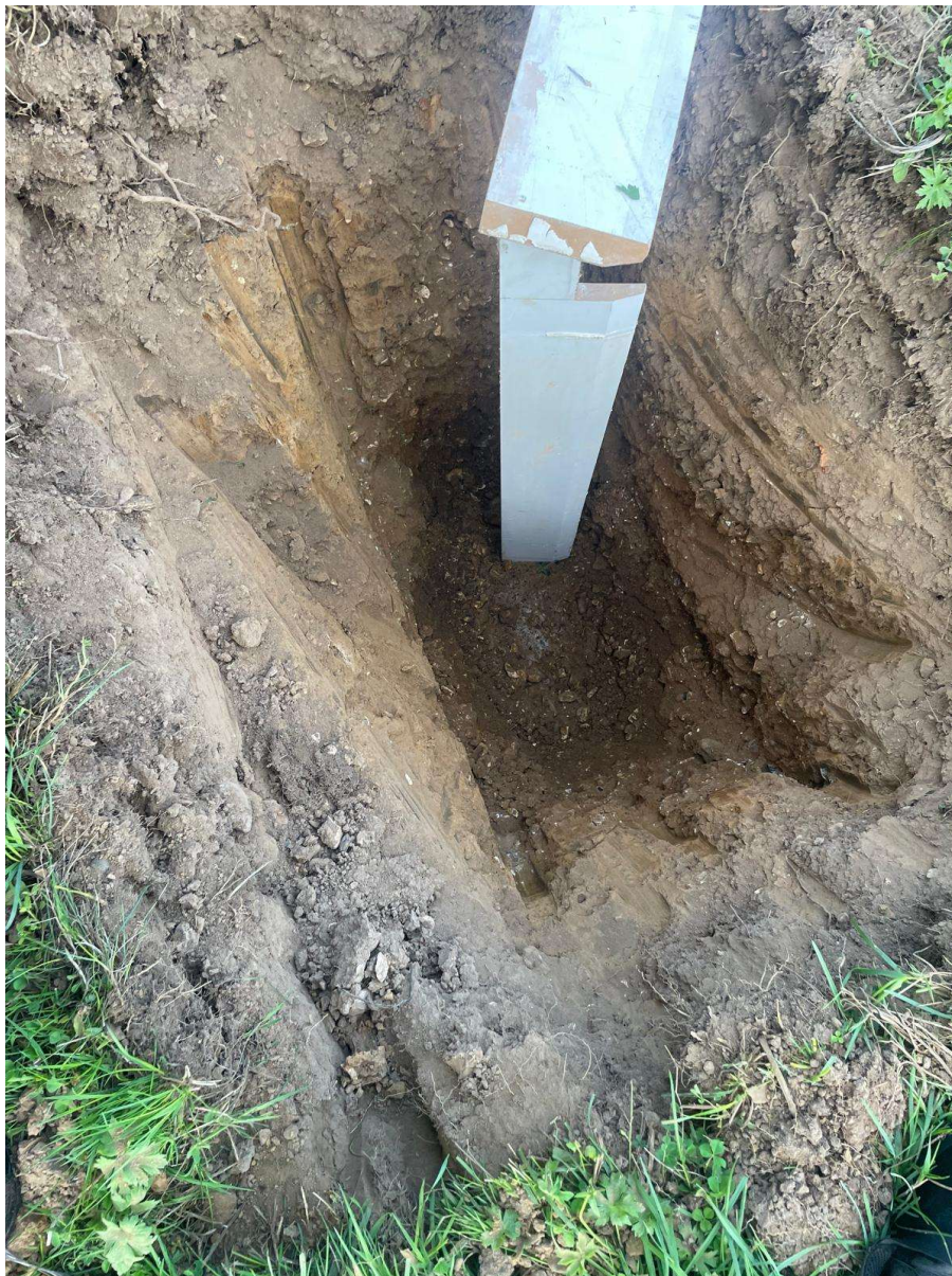
Photograph 3 - Trial excavation showing the deeper test area formed within the lower gravel horizon. The maximum local excavation depth was approximately 1.30 m below ground level and no groundwater was observed before infiltration testing.
