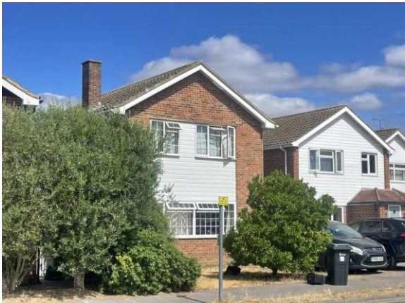
B1 - south-western elevation
