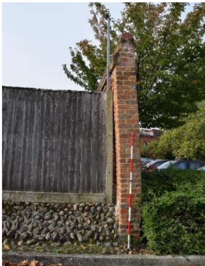
Figure 2. View of Wall H1 (eastern end)
