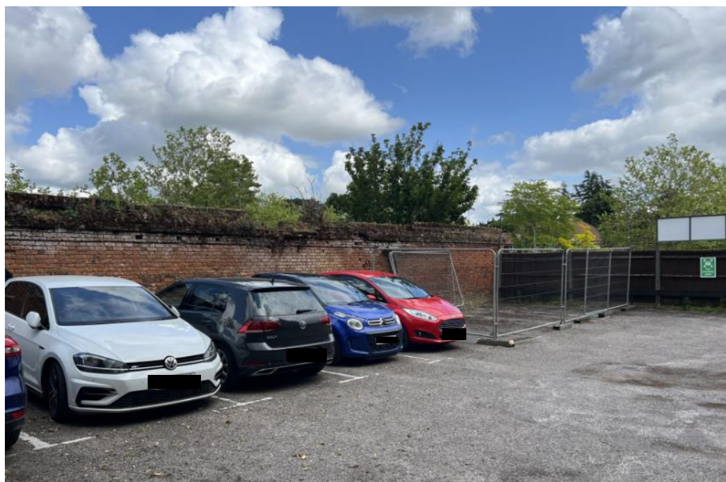
Figure 3. View of Wall H1 (south-eastern elevation)
