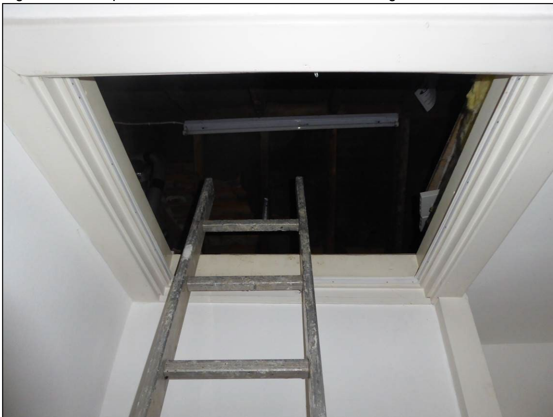
Figure 13. Example of loft hatch. 220 London Road, Wokingham, 05.07.24
