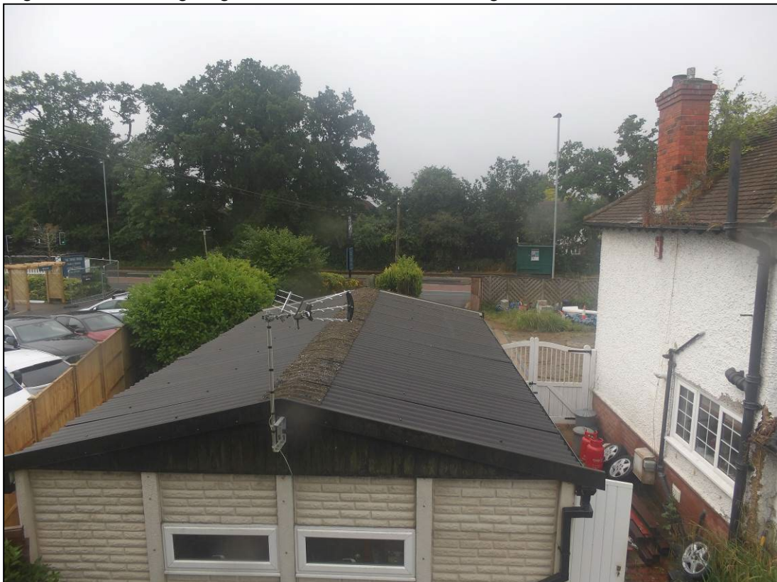
Figure 12. Roof of garage. 220 London Road, Wokingham, 05.07.24
