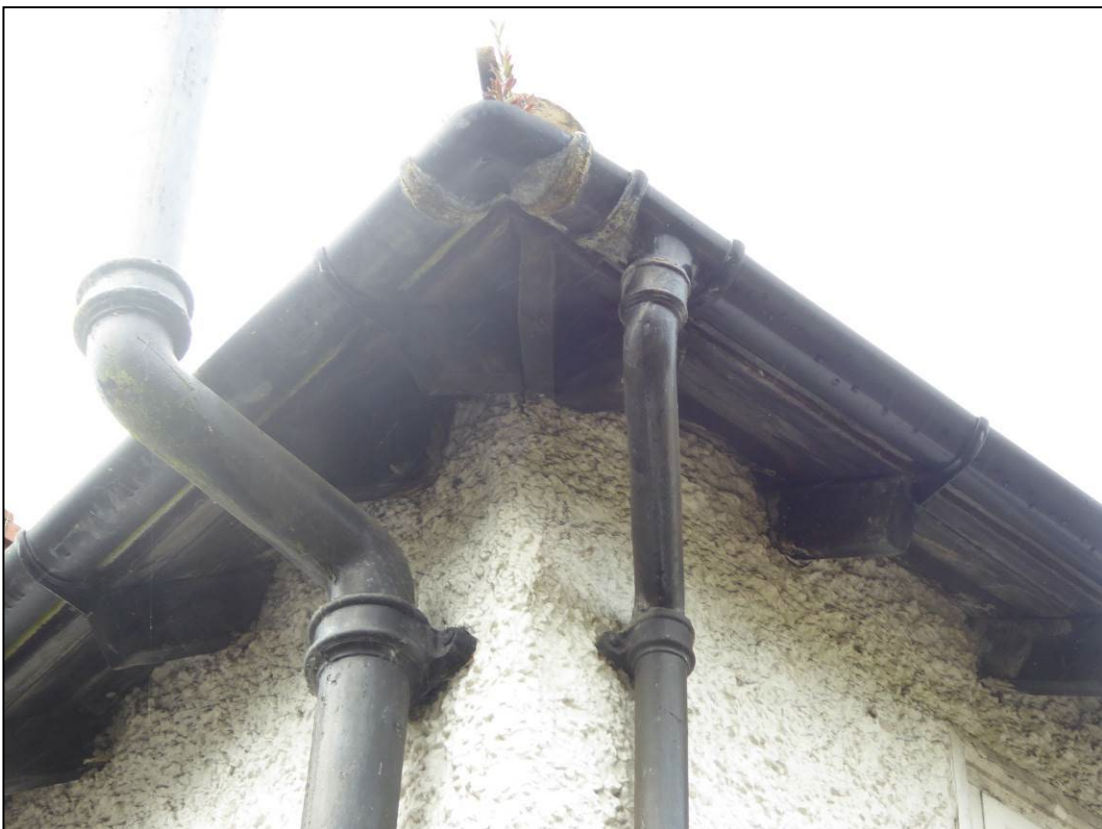
Figure 10. Example of soffits and fascia's. 220 London Road, Wokingham, 05.07.24
