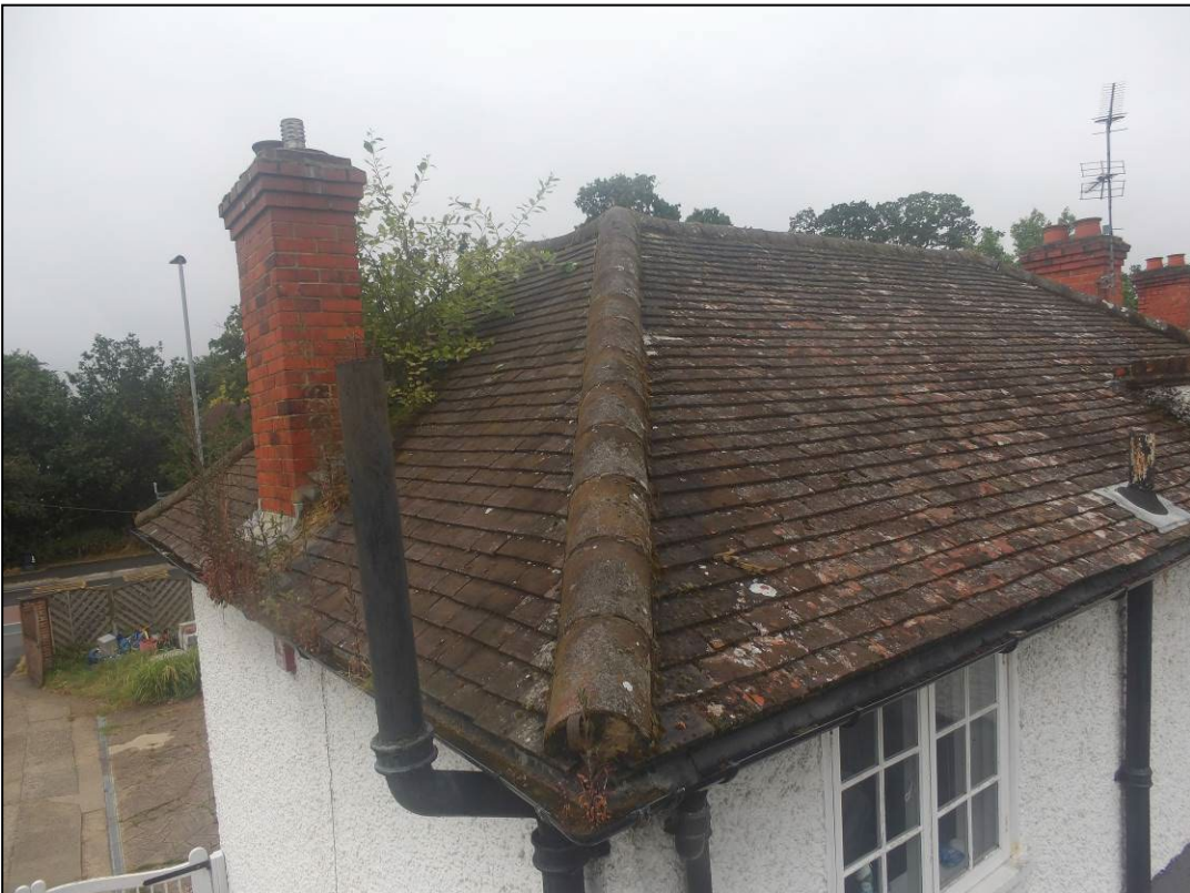
Figure 8. Example of hip tiles. 220 London Road, Wokingham, 05.07.24
