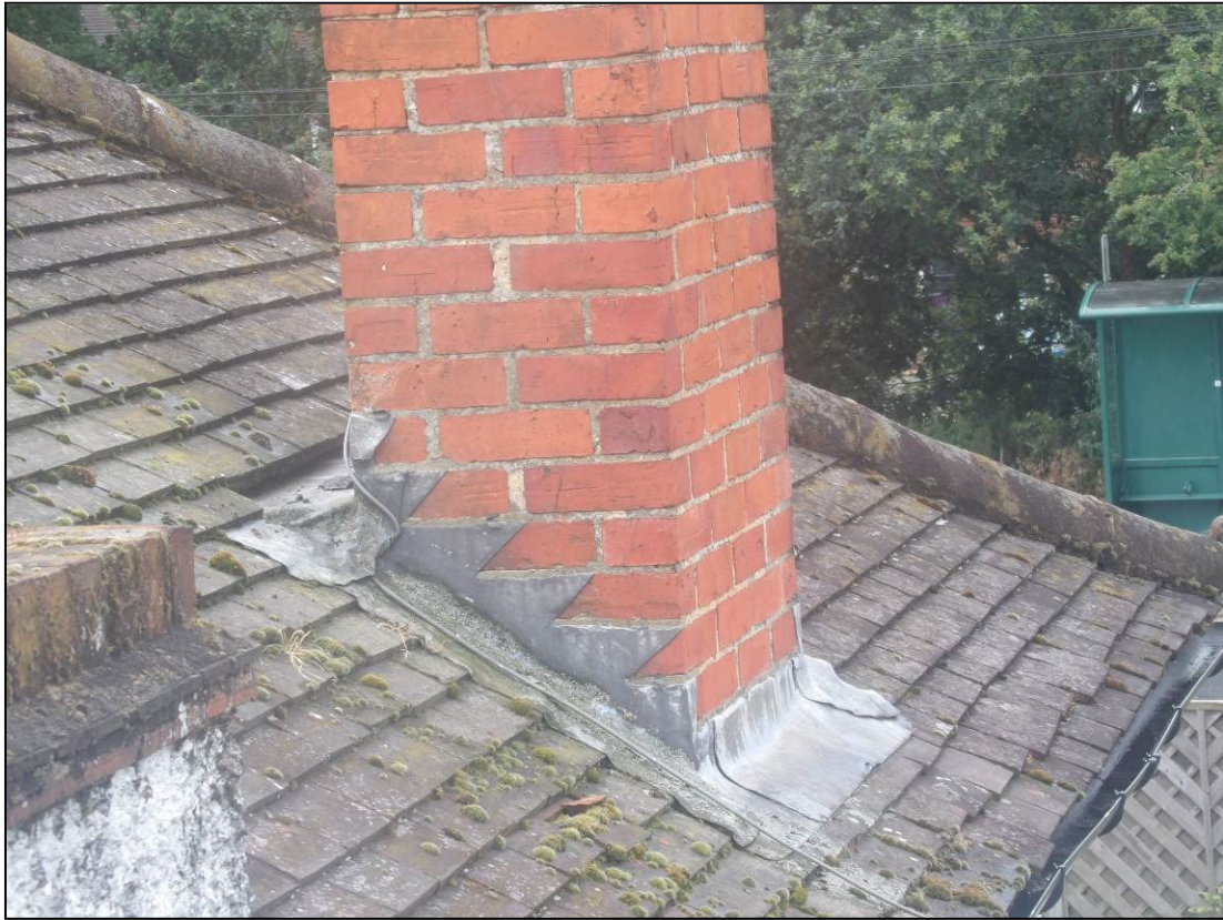
Figure 9. Lead flashing around the chimney. 220 London Road, Wokingham, 05.07.24
