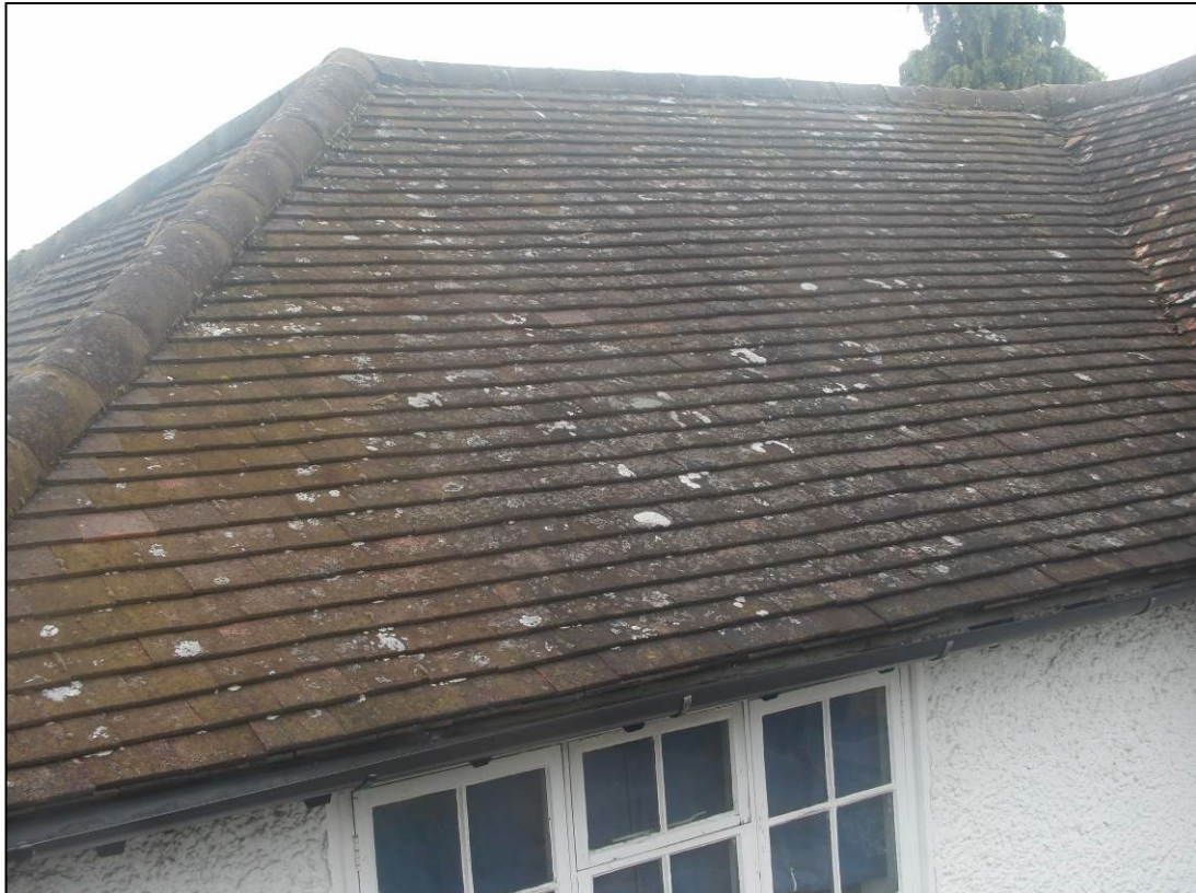
Figure 6. Example of roof tiles. 220 London Road, Wokingham, 05.07.24
