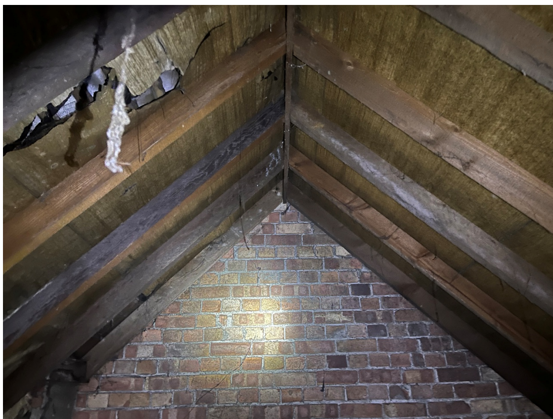
Figure 7. House loft looking west
