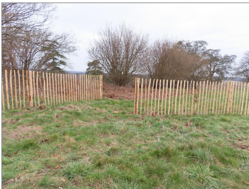
Figure 9, a hit and miss gap to allow for access
