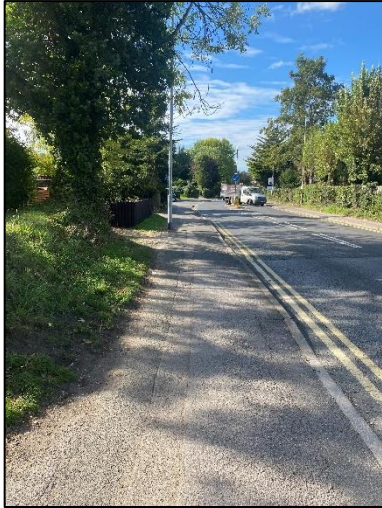
Photograph 3: Footway on Barkham Road (southern extent)
