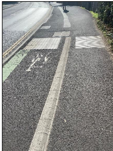
Photograph 18: Segregated footway/cycleway on Wellington Road
