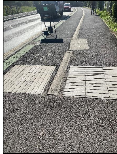
Photograph 17: Segregated footway/cycleway on Wellington Road
