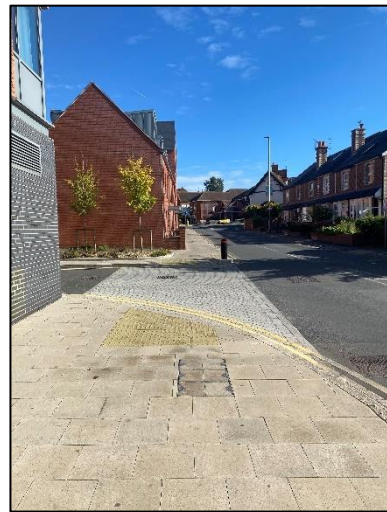
Photograph 25: Footway on Denmark Street
