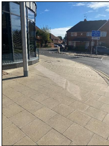
Photograph 24: Widened footway on Wellington Road by roundabout
