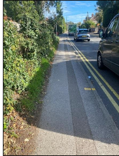
Photograph 4: Footway on Barkham Road (northern extent)
