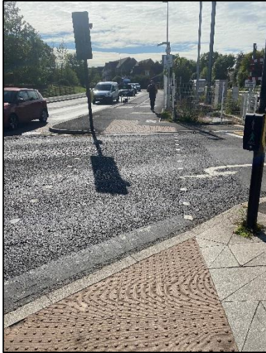
Photograph 16: Signalised pedestrian crossing on Barkham Road (east of level crossing)
