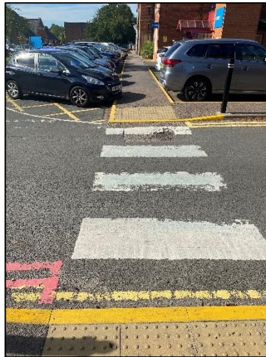
Photograph 8: Pedestrian crossing in Wokingham Hospital car park
