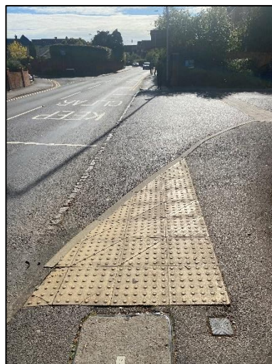
Photograph 20: Pedestrian crossing at Outfield Crescent/Wellington Road junction
