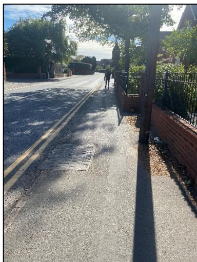
Photograph 19: Footway along Wellington Road
