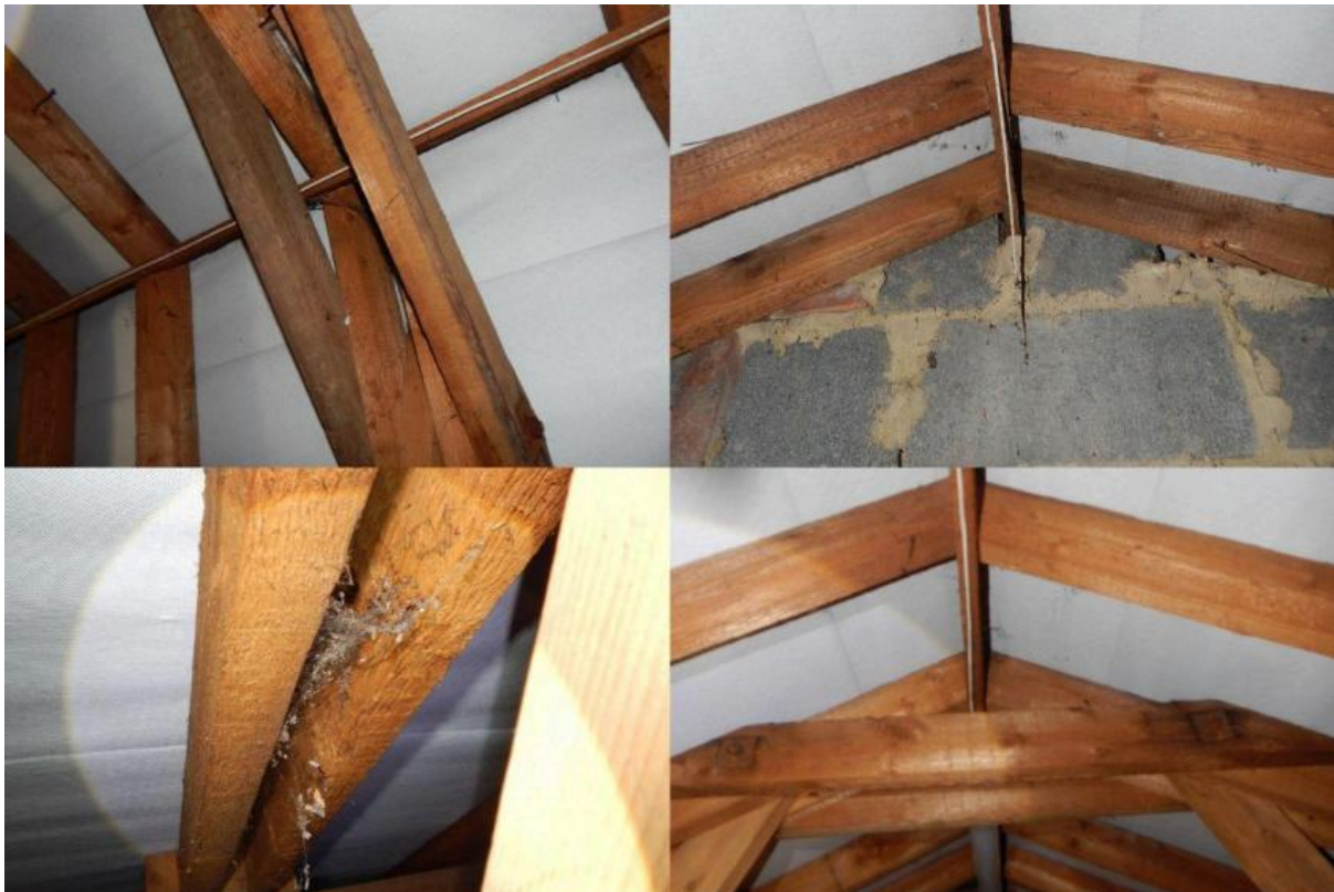
Image 10 – Internal view from within the main upper roof void spaces of the property
