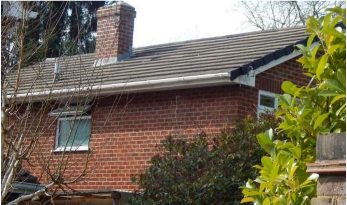
Image 3 – South facing elevation of the property
