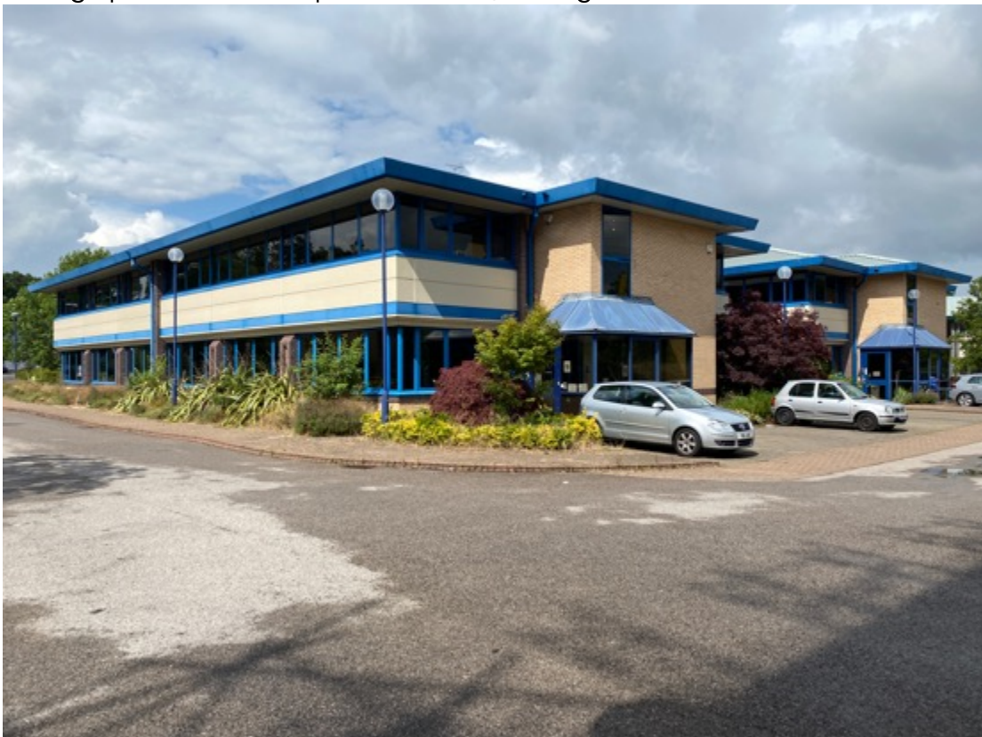
Photograph 2: Southern aspect of the site, looking east
