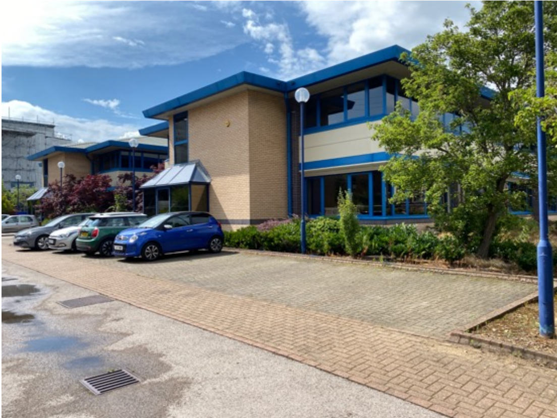
Photograph 1: Southern aspect of the site, looking west
