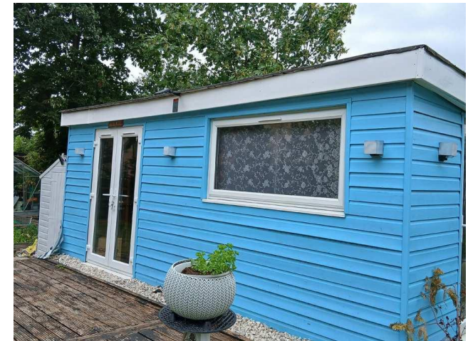
Southern elevation of B2.
