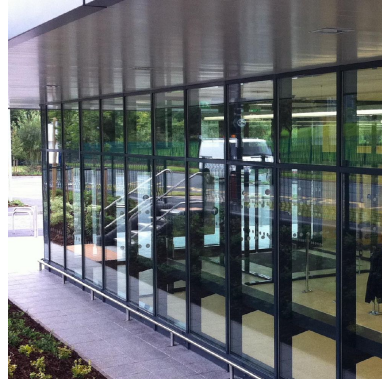
3 Shopfront / entrance / window frames - polyester powder coated aluminium, colour - dark grey ral 7016 (anthracite)
