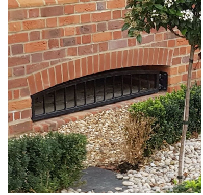
5 Example image of removable protection bars over opening under slab void - Rectangular opening with galvanised steel finish
