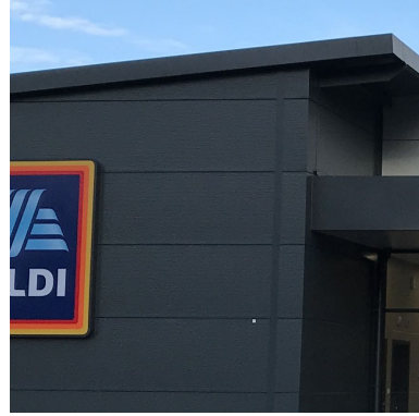
2 Wall - Kingspan KS1000MR anthracite grey cladding RAL 7016
