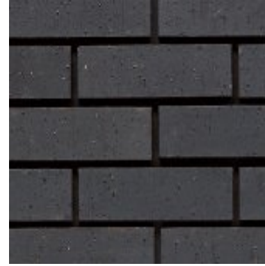
4 Blockleys brick Ltd. 'smooth black' with tarmac y14 (black) to building plinth
