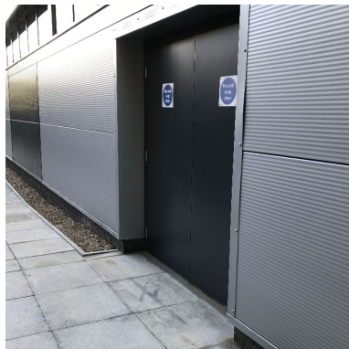
6 External escape doors and frames, steel polyester powder coated finish, colour - dark grey ral 7016 (anthracite)
