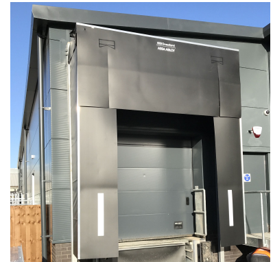
10 Sectional overhead loading bay door - pvf coated steel, ral 7016 (anthracite). Curtain Dock Shelter, colour black
