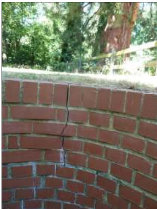
Photograph 2: Vertical crack, north west side, South Lodge, 30.6.2015.
