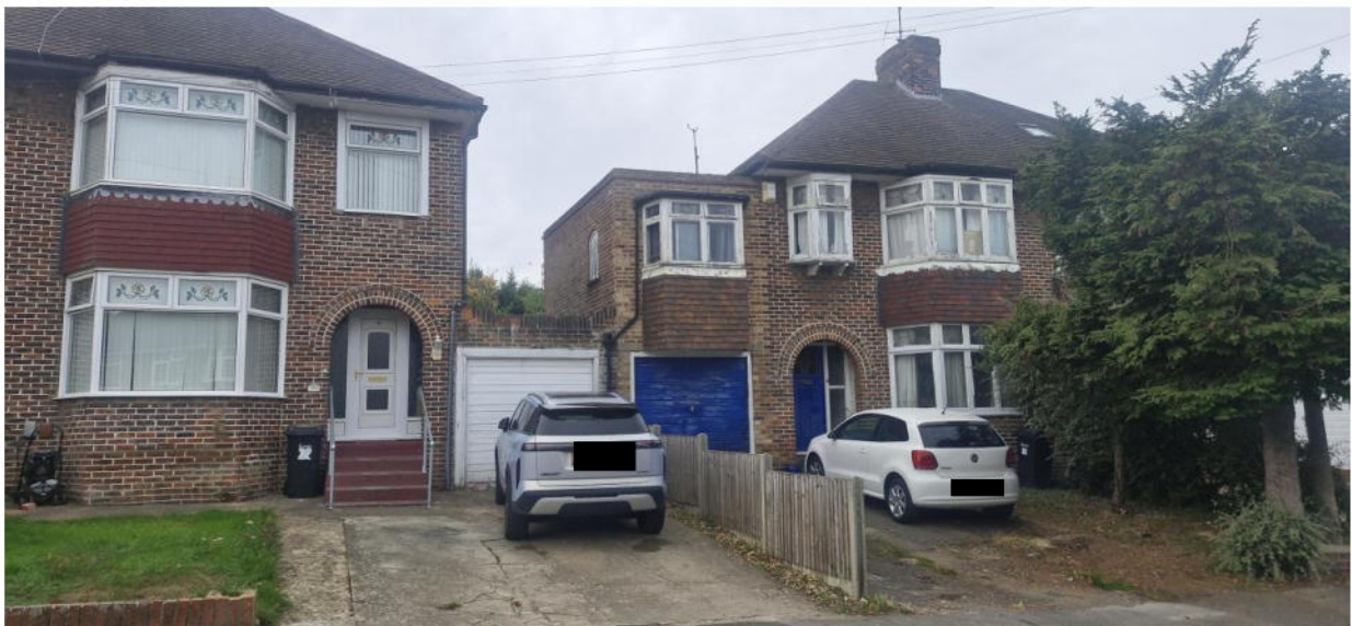
Photo 5: flat roof two storey side extension at No.20
