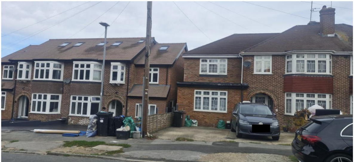
Photo 7: gable end two storey side extension at No.9
