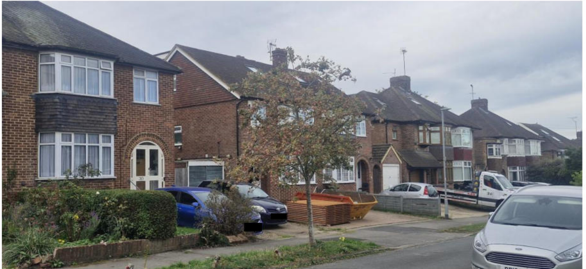
Photo 2: side elevation of No.28, with gable end roof
