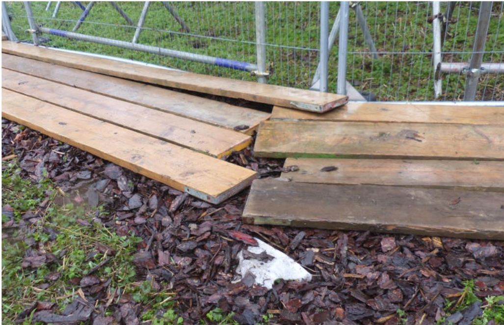
Fig 3. Scaffold boards on top of wood chips serving as ground protection. Note the geotextile layer underneath
