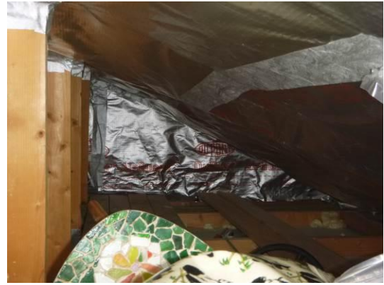
Photograph 12. Intact foil lined roofing felt across roof and gable end (roof void).
