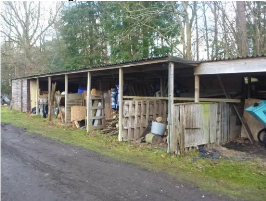
Photograph 5. Sheds, car port and log stores to the south-east of the property, viewed from the north.
