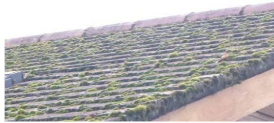
Photograph 7. Tight ridge tiles and intact mortar (south elevation).
