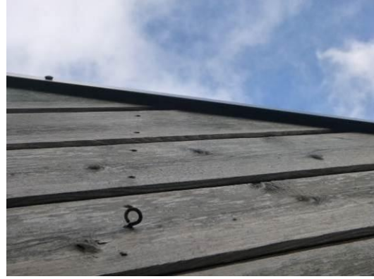
Photograph 15. Metal flashing tight to timber cladding on detached office (eastern elevation).
