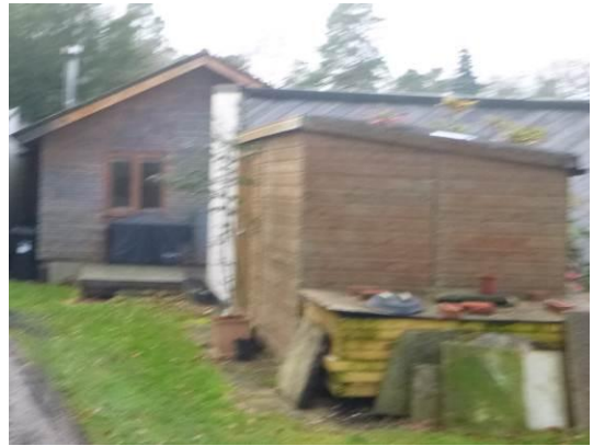
Photograph 4. Detached office and timber storage shed, viewed from the east.
