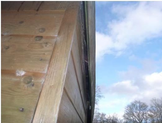
Photograph 16. Timber bargeboard tight to timber shed (eastern elevation).
