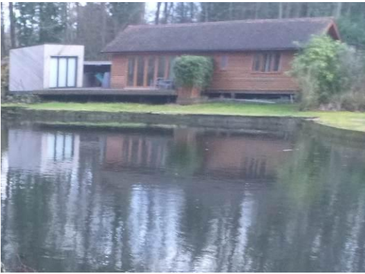
Photograph 3. Rear of the property and detached office building, viewed from the north.
