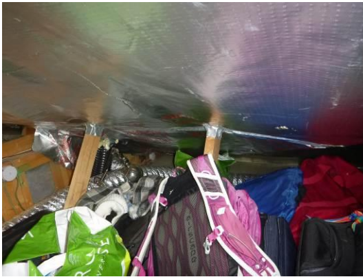
Photograph 13. Roof void of pre-trussed rafter construction.
