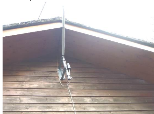
Photograph 9. Timber soffit tight to tongue-in-groove timber cladding along eaves (west elevation).
