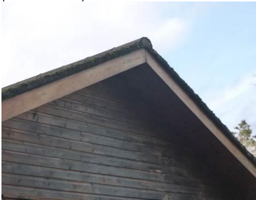
Photograph 8. Intact verge mortar (east elevation).
