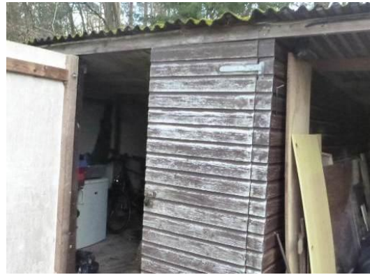
Photograph 17. Intact timber cladding on storage shed (northern elevation).
