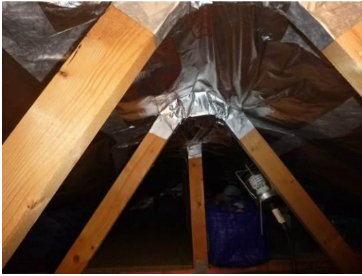
Photograph 11. Roof void of pre-trussed rafter construction.
