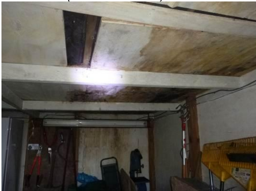
Photograph 18. Intact timber cladding on storage shed (Storage shed internal).
