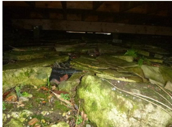
Photograph 14. Rocks present below raised decking.
