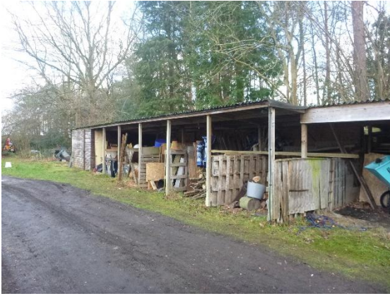
Photograph 3. Storage sheds and log stores along the southern side of the site.
