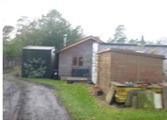
Photograph 2. Driveway, detached dwelling and timber shed viewed from the west.
