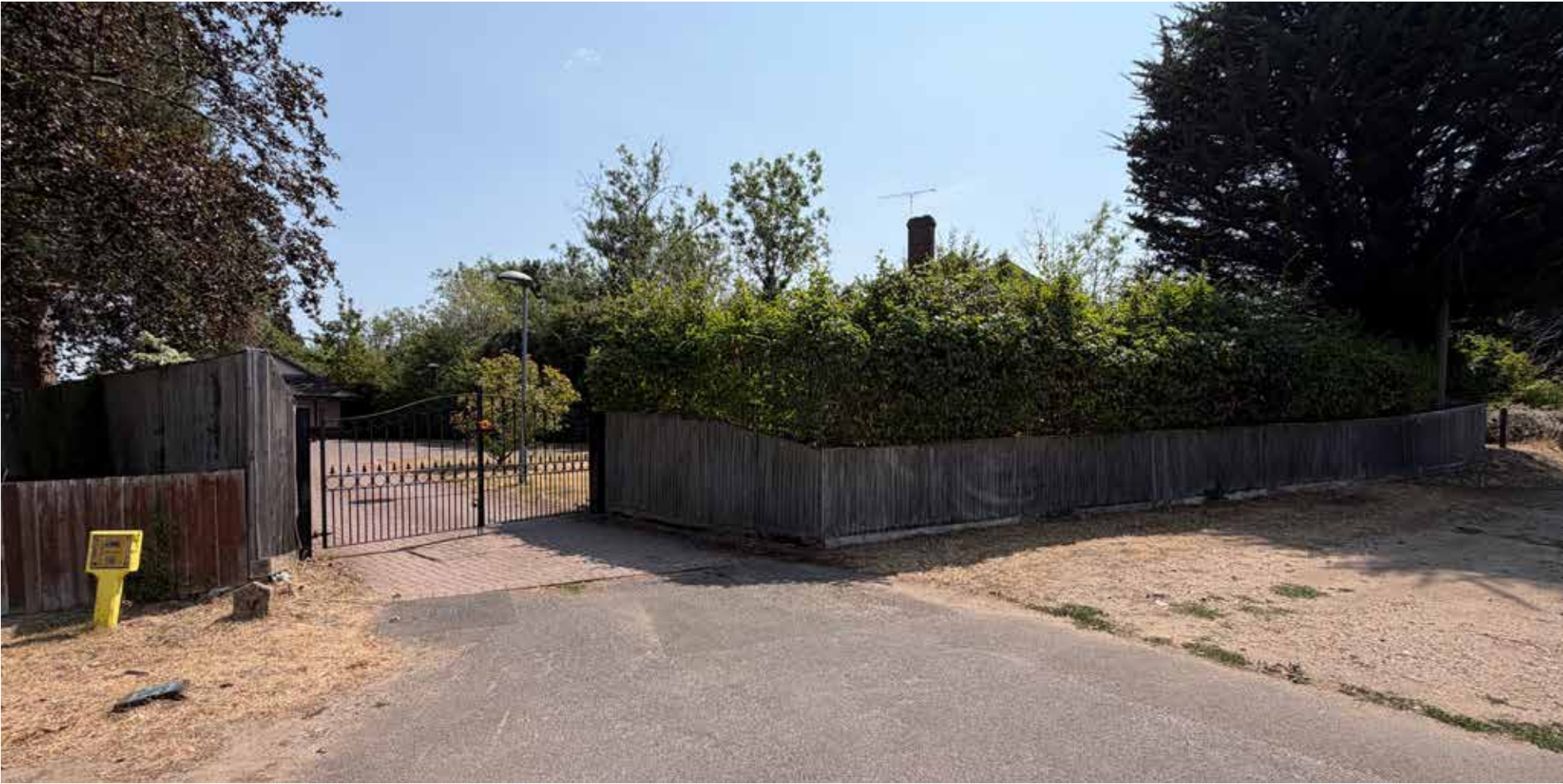
Existing front boundary of 20 Pitts Lane
