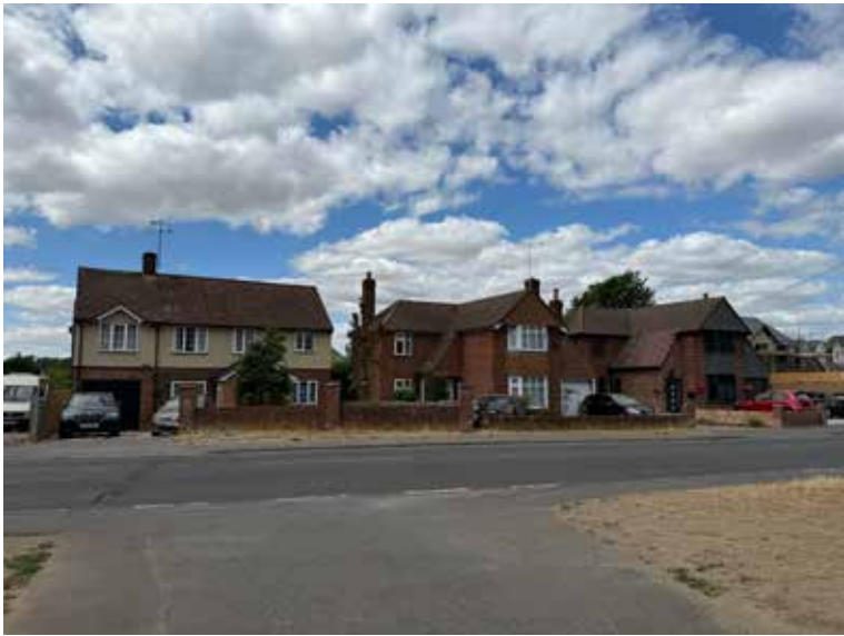
No.27, 29, 31 and recently extended no. 33 Pitts Lane (Opposite Context)
