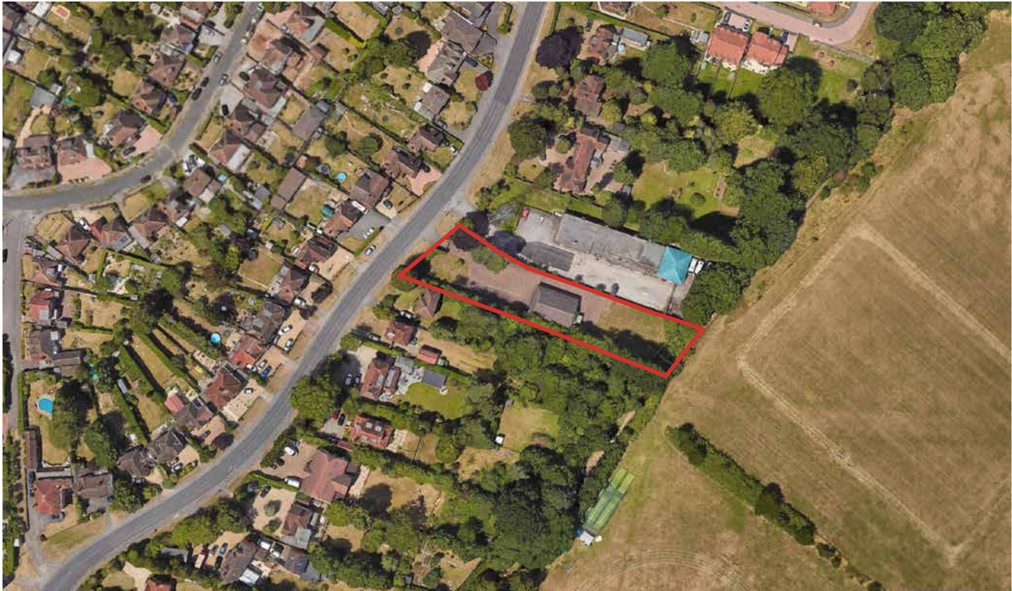
Aerial view of site and context with 20 Pitts Lane outlined in red
