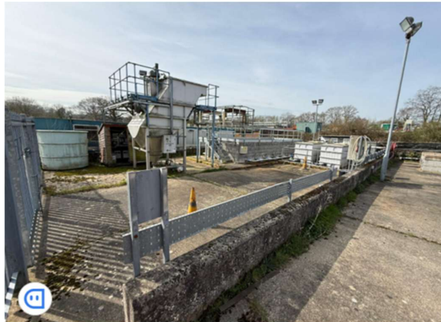
Photograph 7– Disused R&D Compound Area
