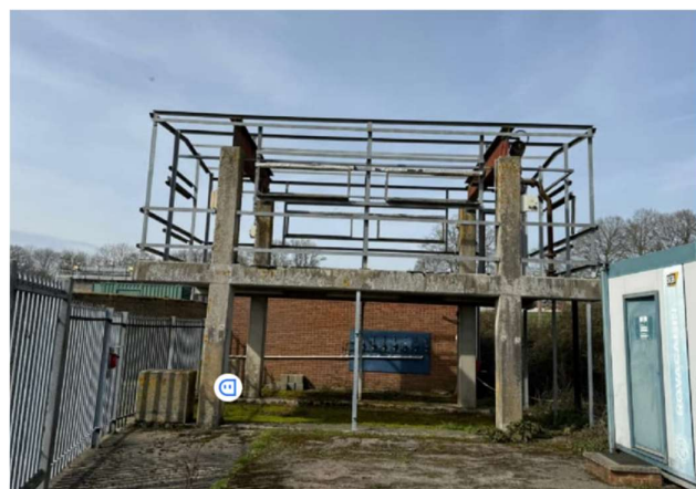
Photograph 9– Disused concrete frame inside R&D Area
