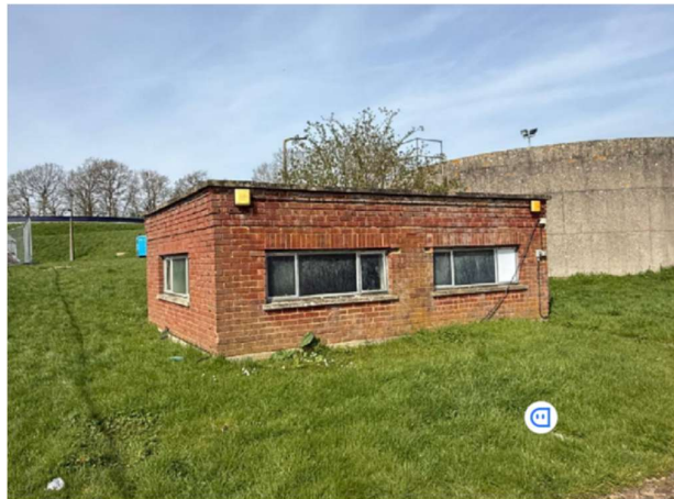
Photograph 1 – Disused Sludge Pumphouse Building
