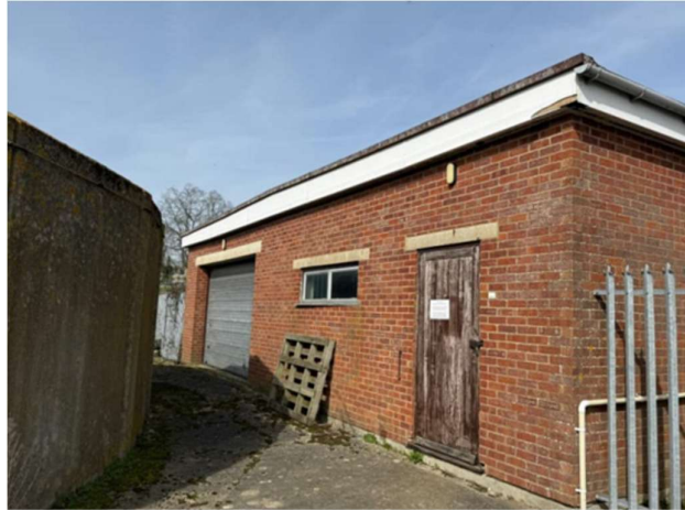
Photograph 10 – Disused R&D Workshop
