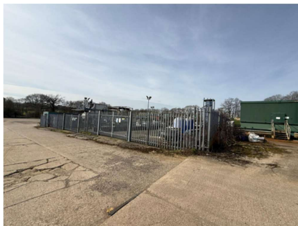
Photograph 6– Disused R&D Compound Area
