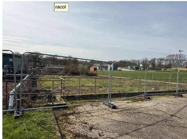
Photograph 4– Sludge Drying Beds
