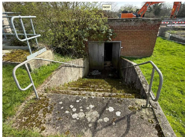
Photograph 2 – Disused Sludge Pumphouse Building Access
