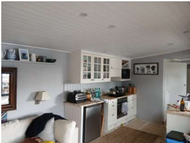
Plate 5: Sloping ceiling in northern portion of cabin
