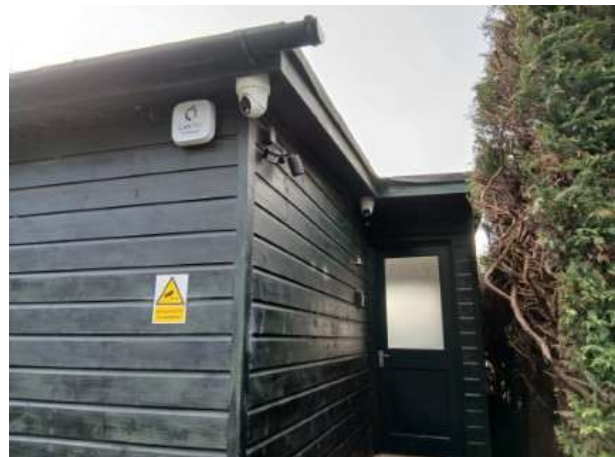
Plate 2: Covered porch on north corner of cabin
