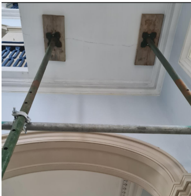
Underside of cantilevered landing of stairs at first floor.
