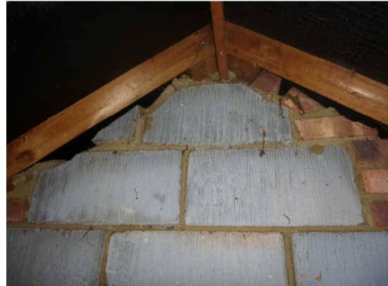
Photograph 20. Gable ends of blockwork construction with sections of brickwork (loft void).
