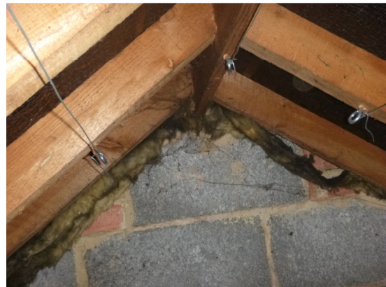
Photograph 22. Fiberglass between timber rafters and blockwork of previous external wall (roof void).
