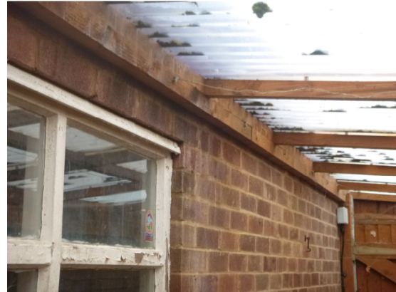
Photograph 4. Sloping canopy connecting the eastern side extension as viewed from south.
