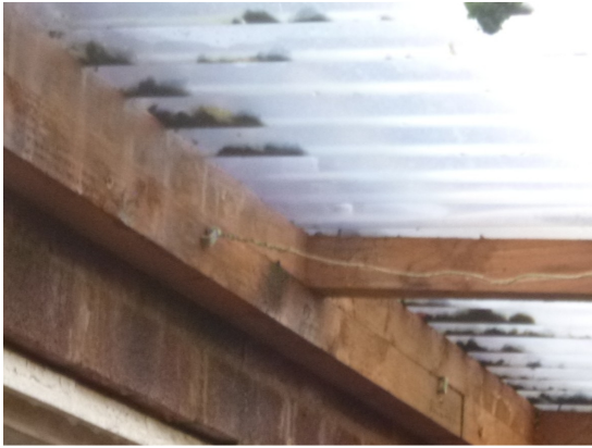
Photograph 9. Plastic sheeting roof of the sloping canopy was intact and the timber frame tight to brickwork of side extension (eastern elevation).
