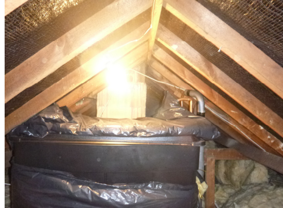
Photograph 16. Loft space viewed from loft hatch and large covered water tank (roof void).
