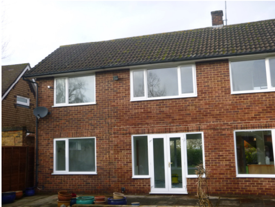
Photograph 3. Rear of house viewed from south
