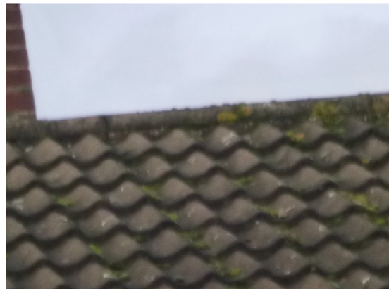
Photograph 6. Ridge tiles tightly mortared to interlocking roof tiles (rear elevation).
