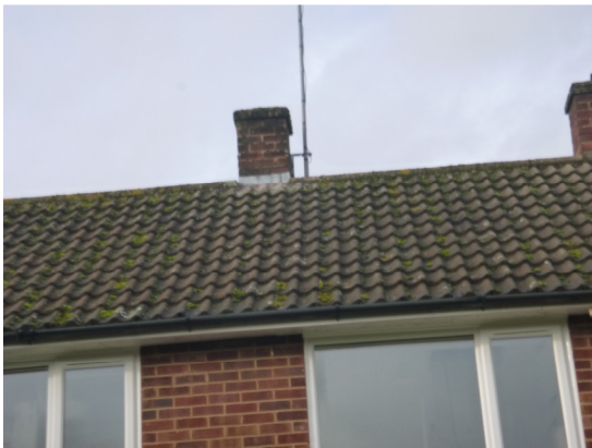
Photograph 5. Intact/tight interlocking roof tiles on the rear elevation.
