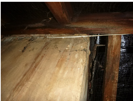
Photograph 23. Rendered brick chimney with small gaps exposing external interlocking roof tiles (roof void).
