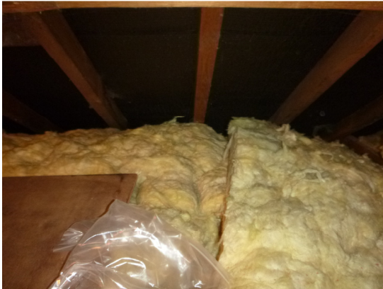
Photograph 19. Fibreglass insulation between the timber joists (roof void).
