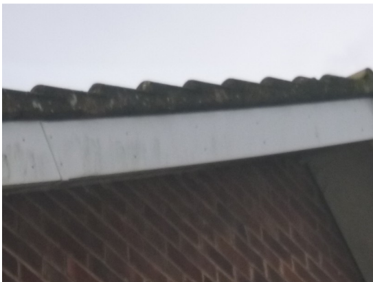
Photograph 7. Verge mortar intact (western elevation).
