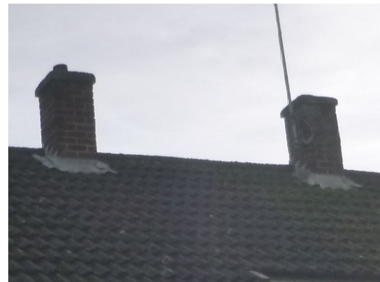
Photograph 8. Lead flashing around both chimneys tight to roof tiles (front elevation).
