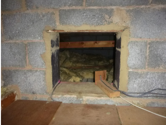
Photograph 15. Gap in previous external wall into second section of roof void (roof void).
