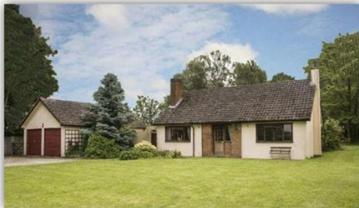
Brandywell House and Garage - Front View
