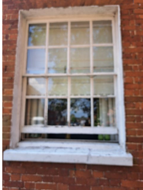
Photo 18 – Ground floor front window LHS
