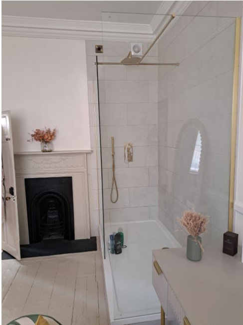
Photo 24 – First floor bathroom
