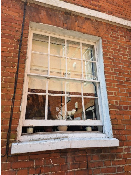
Photo 17 – ground floor front window RHS
