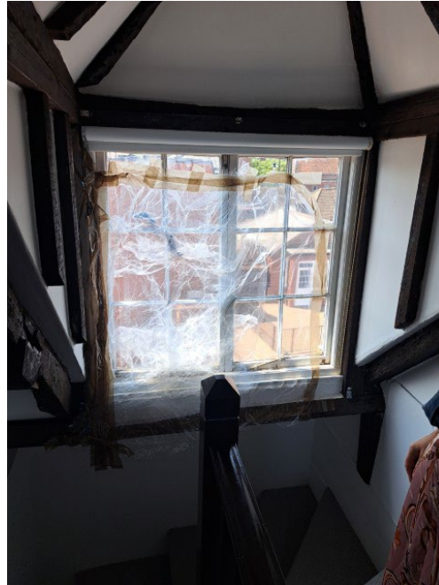
Photo 15 – third floor rear window
