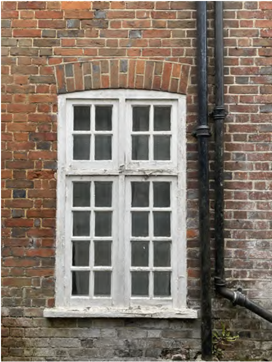
LGW-09 Existing condition
