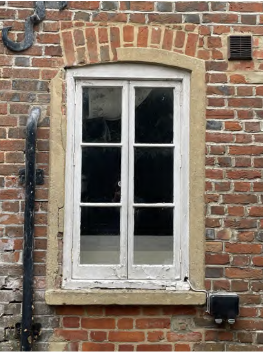
LGW-08 Existing condition
