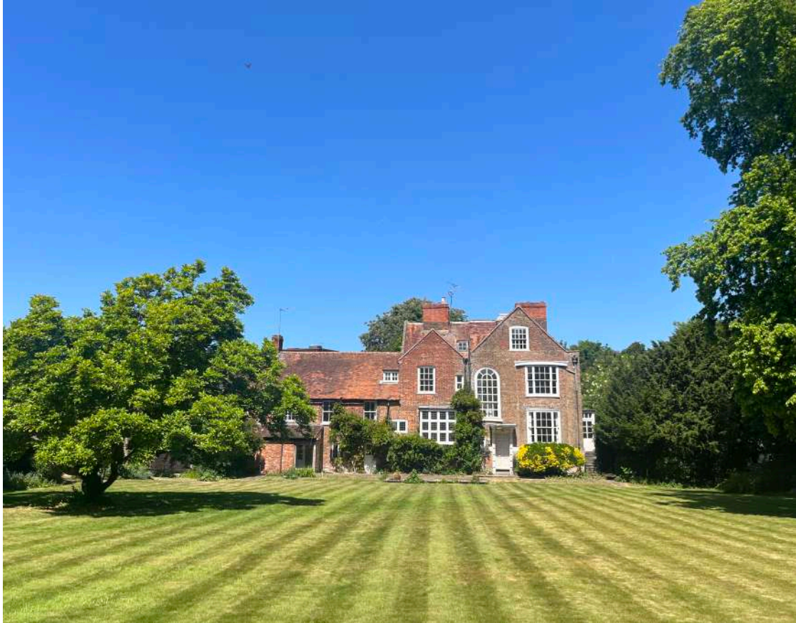
Bird Place - Existing rear facade (south)
