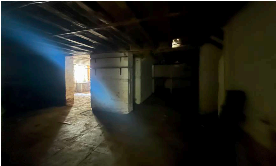
Existing basement - View 1
