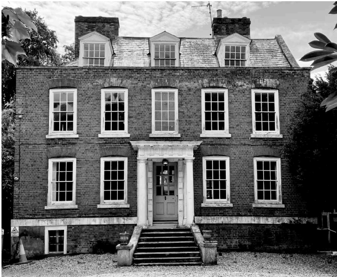
Bird Place – Existing front facade (north)
