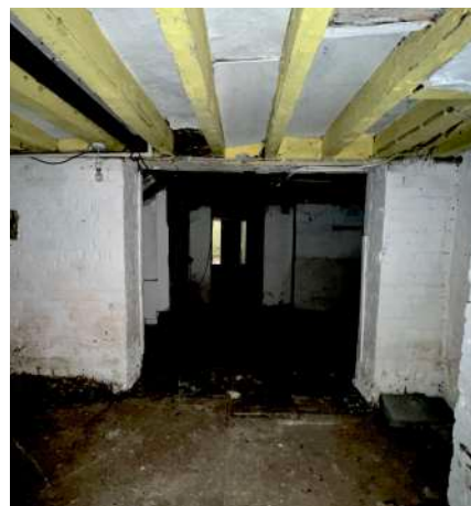
Existing basement - View 3
