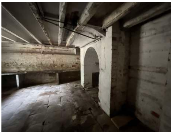
Existing basement - View 2
