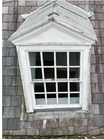
Slate tiles to front roof
