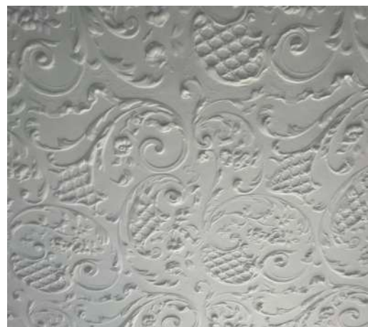
Ground floor ceiling detail
