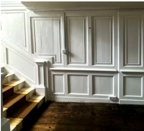
Existing wall panelling to entrance hall
