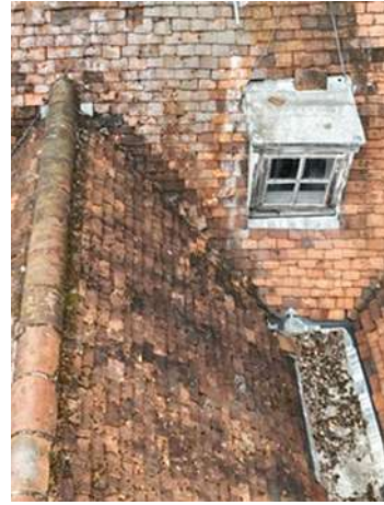
Clay tiles to rear roof pitches
