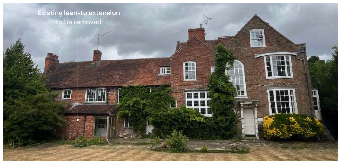
Bird Place - Existing rear facade (south)
