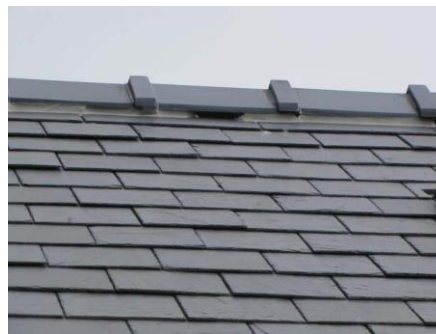
Access feature created from a gap in the mortar
