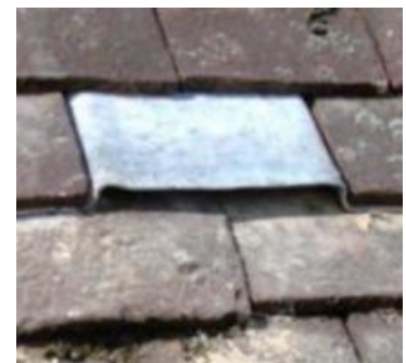
DIY of a bat access feature in lead
