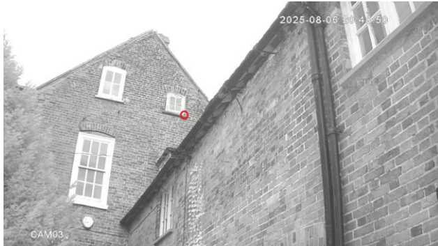
First soprano pipistrelle bat seen emerging on the infrared camera during the second survey
