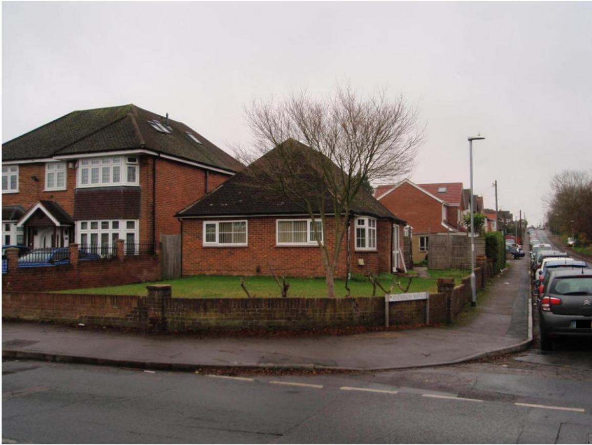
Current view from Culver Lane/Anderson Avenue
