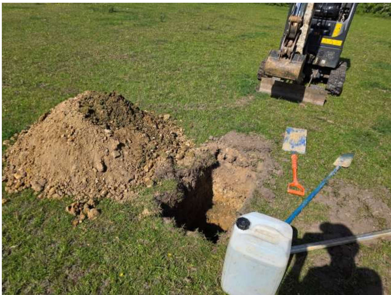
Figure 2 - SW1 during excavation
