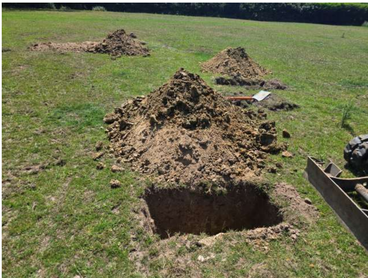
Figure 7 - GW1 during excavation
