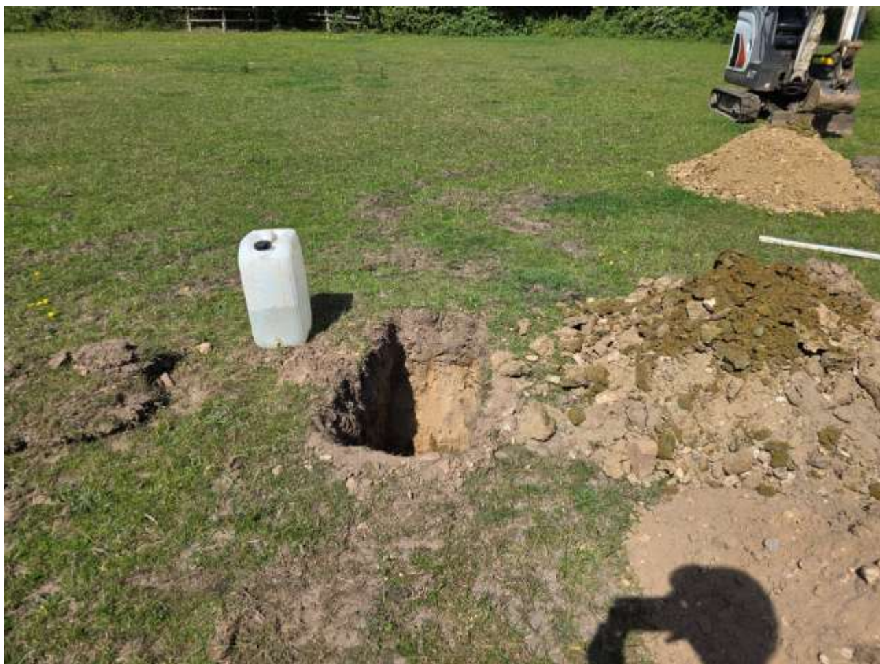
Figure 5 – Soakaway pit 2 during excavation
