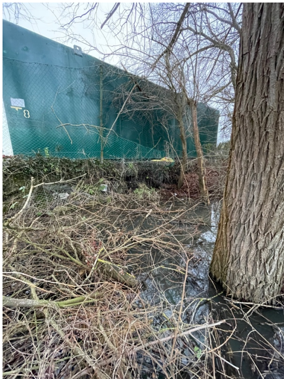
Photograph illustrating subsiding flood water up to site boundary and the unretained made ground on which the site stands with fuel tanks in situ
