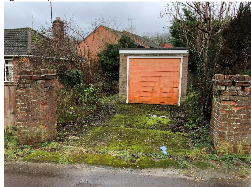
Fig 13. Garage of Jalno, Norton Road.
