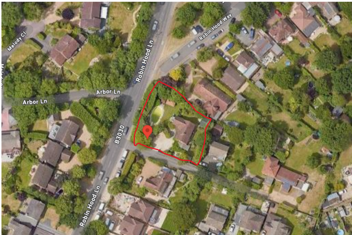
Figure 02. Aerial view of site (highlighted red)
