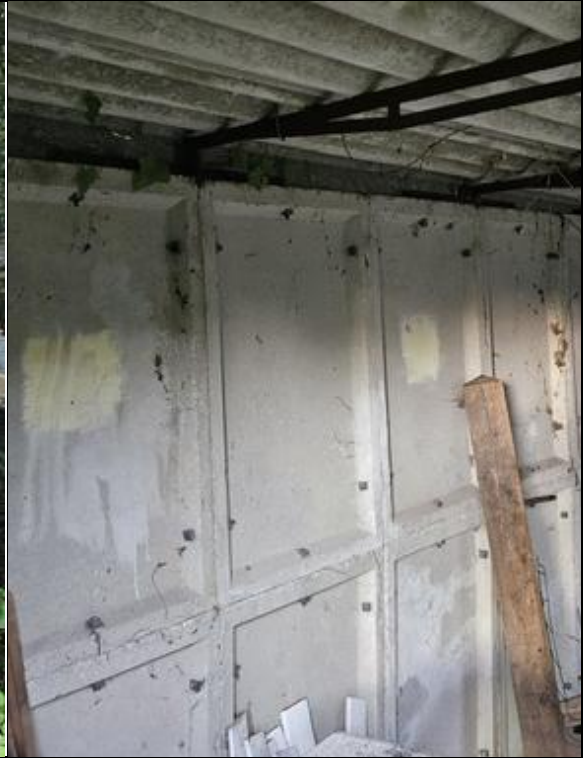
Photograph 6: Garage interior with corrugated metal roofing.
