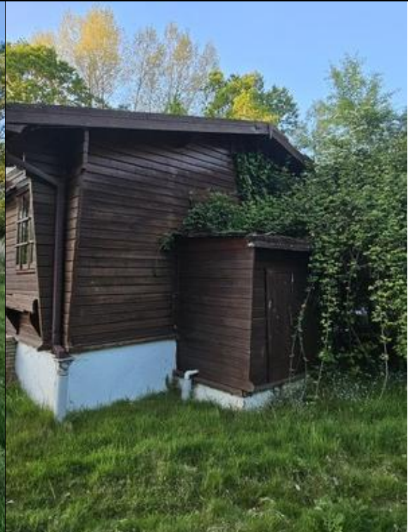
Photograph 14: Wooden clad pool house – negligible potential.
