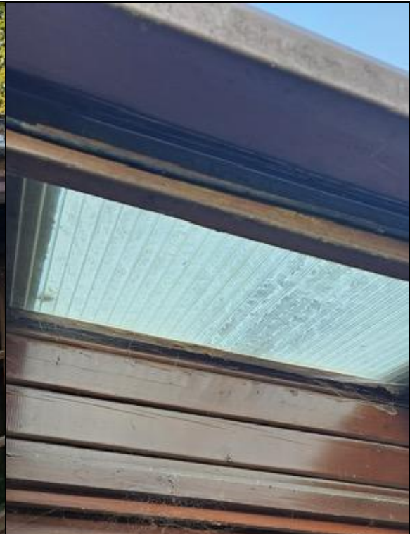
Photograph 18: Pool house skylight.
