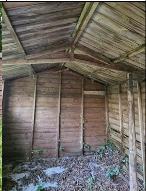
Photograph 4: Interior of Shed outbuilding B.
