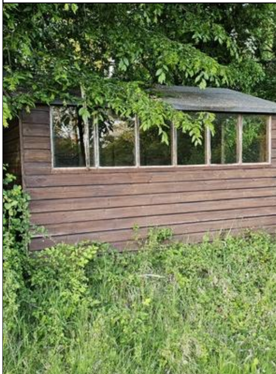
Photograph 3: Shed outbuilding B.
