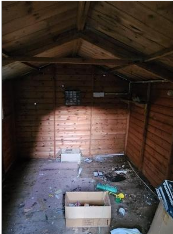
Photograph 1: Wooden shed A interior.
