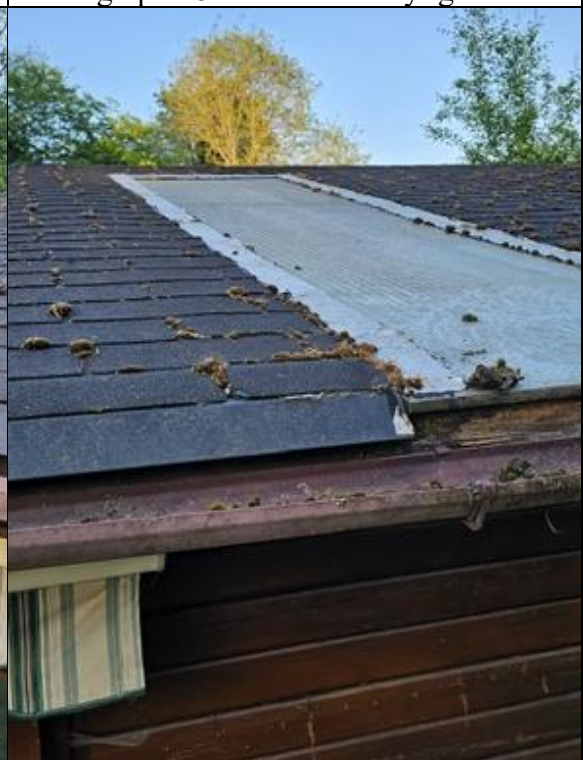
Photograph 20: No gaps in roofing.
