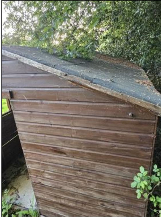
Photograph 5: Simple structure with asphalt roof B.
