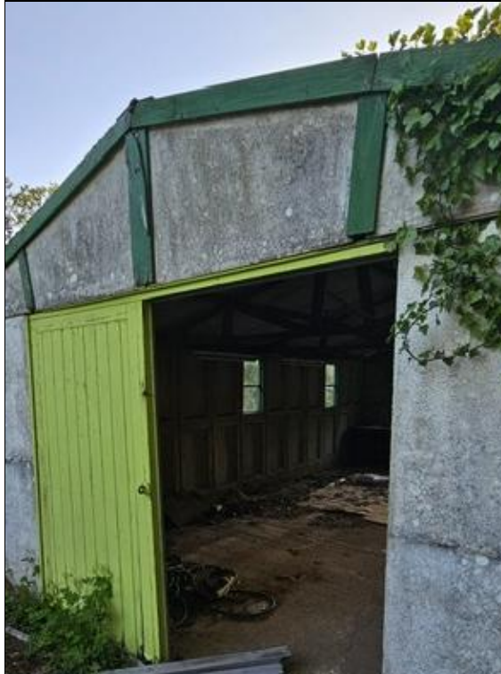
Photograph 11: Front of garage.
