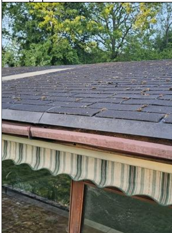
Photograph 19: No gaps in roofing.
