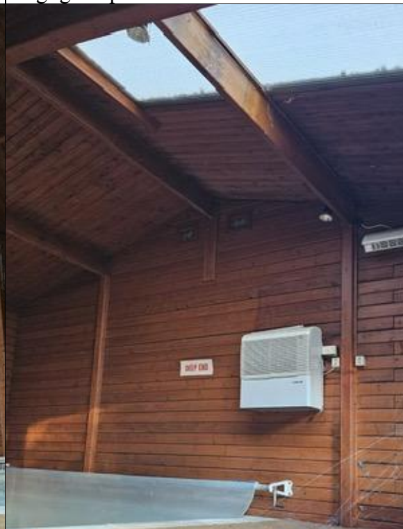
Photograph 16: Pool house interior with skylight.
