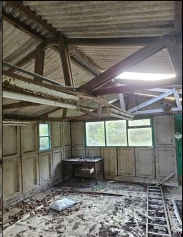
Photograph 10: Garage interior – simple structure with large cavities.
