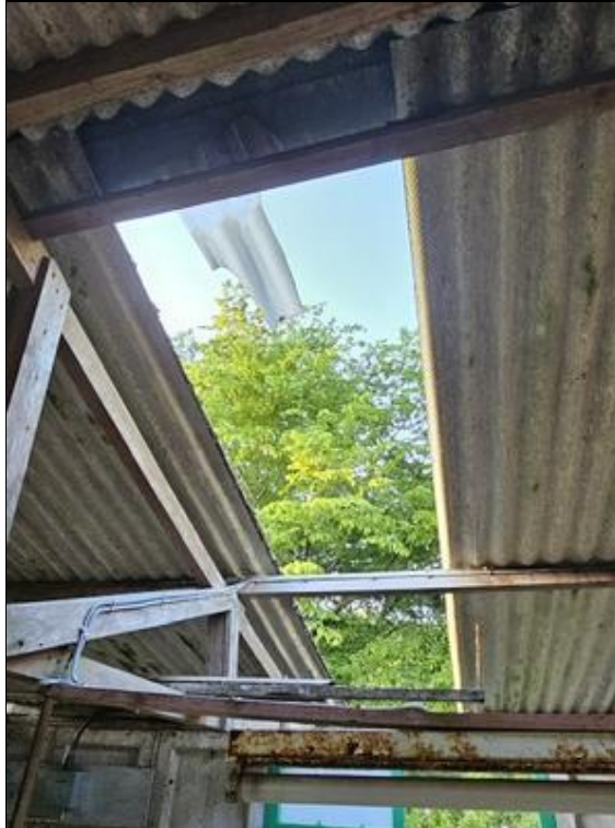
Photograph 9: Garage interior – simple structure with large cavities.
