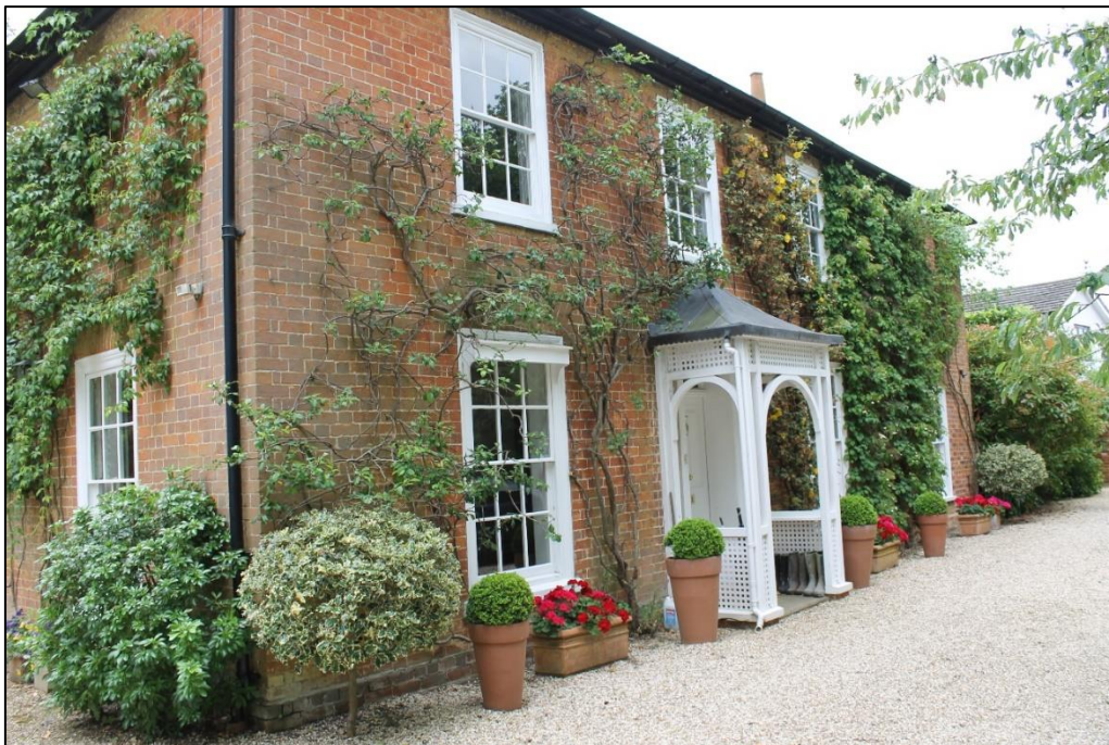
Photograph 1 – Front elevation as viewed from the driveway
