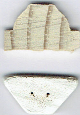
Internal Glazing bar profile
