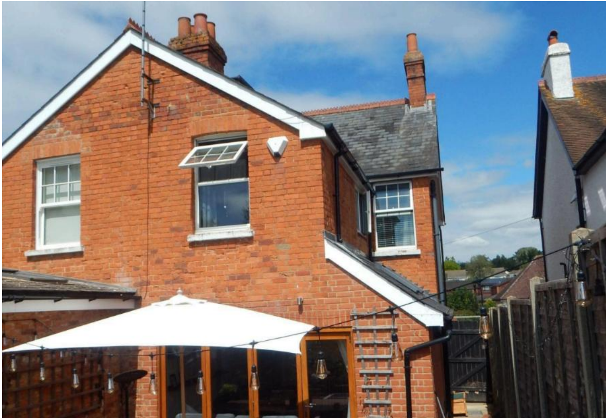
Image 3 – South/East facing elevation of the property
