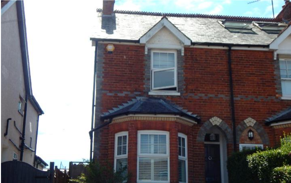
Image 1 – North/West facing elevation of the property
