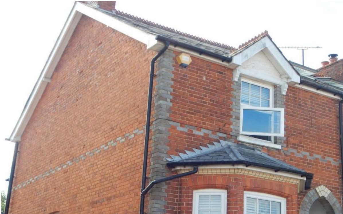
Image 4 – North/East facing elevation of the property
