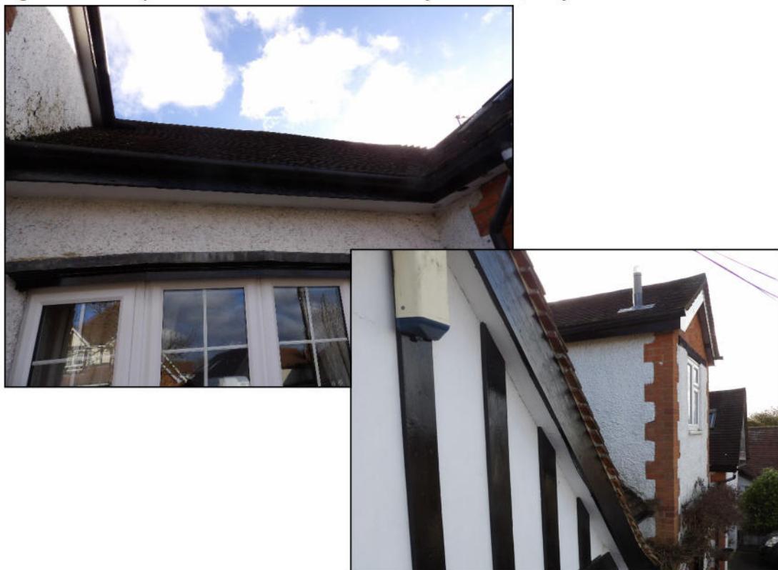
Figure 8. Example sealed soffits/fascias. 30 Byron Road, Twyford. 20.01.26
