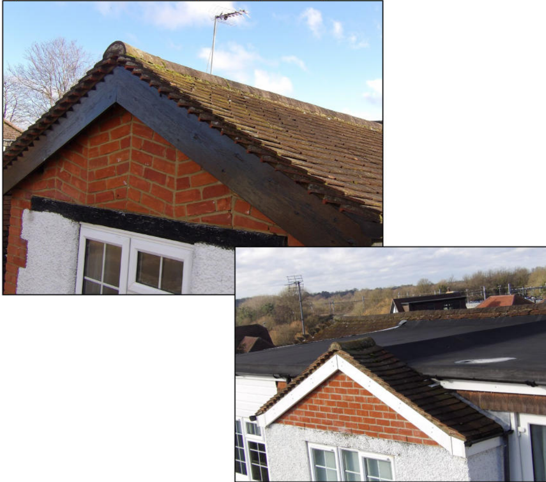
Figure 8. Example sealed soffits/fascias. 30 Byron Road, Twyford. 20.01.26
