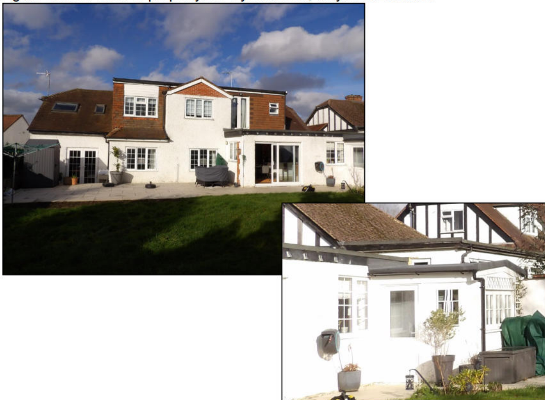
Figure 4. Rear view of property. 30 Byron Road, Twyford. 20.01.26
