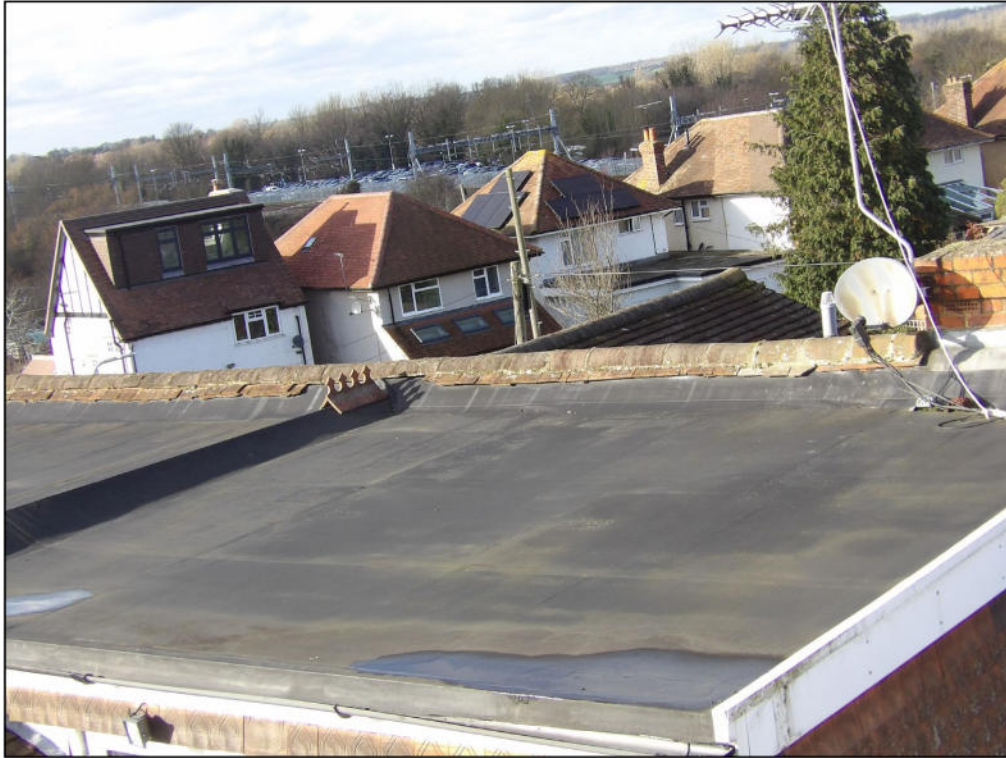
Figure 9. Example well fitted membrane on rear dormer. 30 Byron Road, Twyford. 20.01.26
