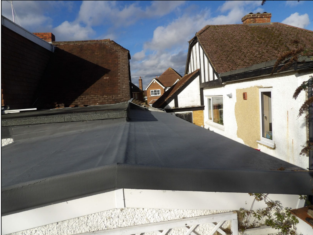
Figure 11. Example bitumen felt and membrane on rear extension. 30 Byron Road, Twyford. 20.01.26
