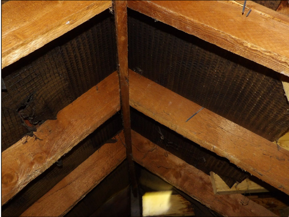
Figure 14. Internal view of torn bitumen felt in remaining loft space. 30 Byron Road, Twyford. 20.01.26
