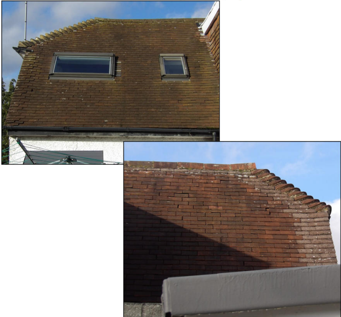
Figure 6. Example sealed ridge tiles. 30 Byron Road, Twyford. 20.01.26
