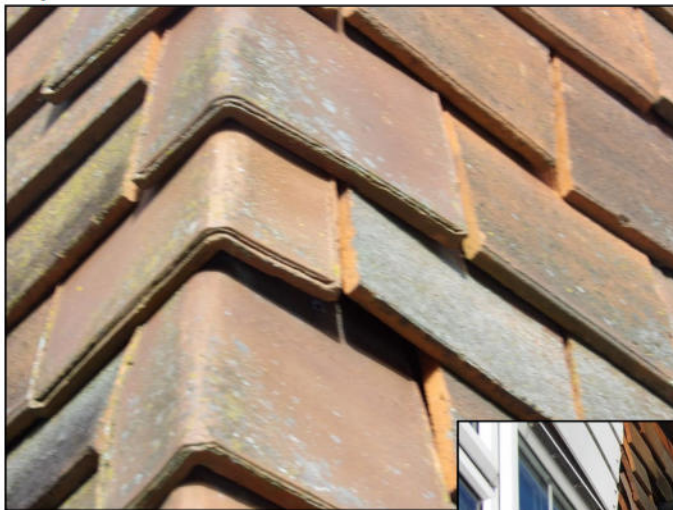
Figure 10. Example moved hanging tiles and gaps on rear dormer. 30 Byron Road, Twyford. 20.01.26
