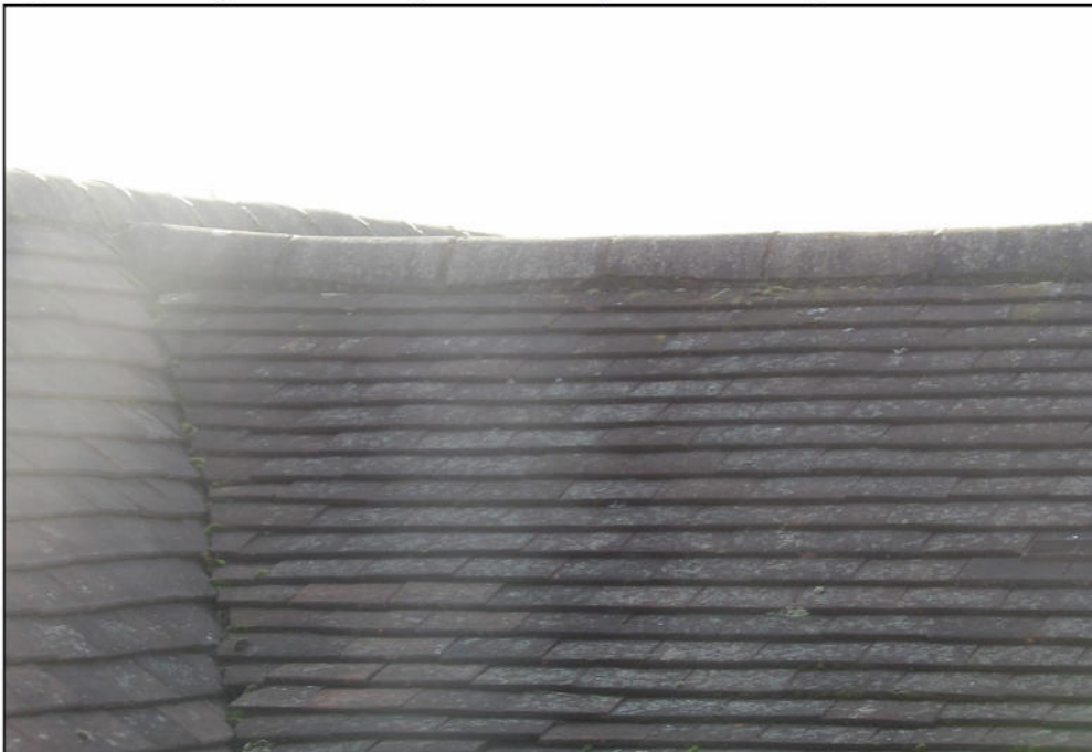
Figure 6. Example sealed ridge tiles. 30 Byron Road, Twyford. 20.01.26
