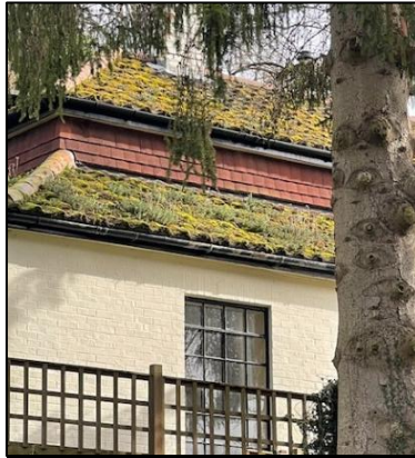
Hanging wall tiles.
