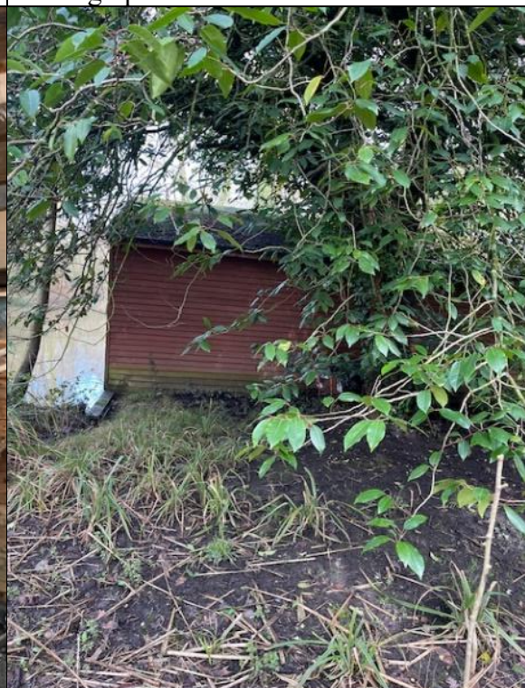
Photograph 26: Boathouse side elevation.
