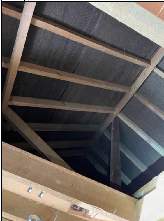
Photograph 21: Liner in the garage loft space.
