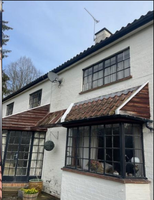
Photograph 10: Wooden cladding above bay window.
