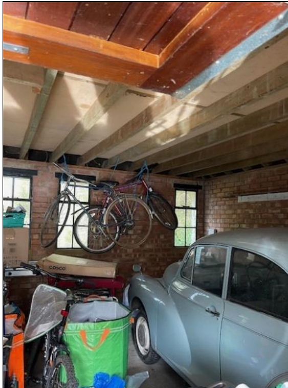
Photograph 19: Garage interior used for storage.
