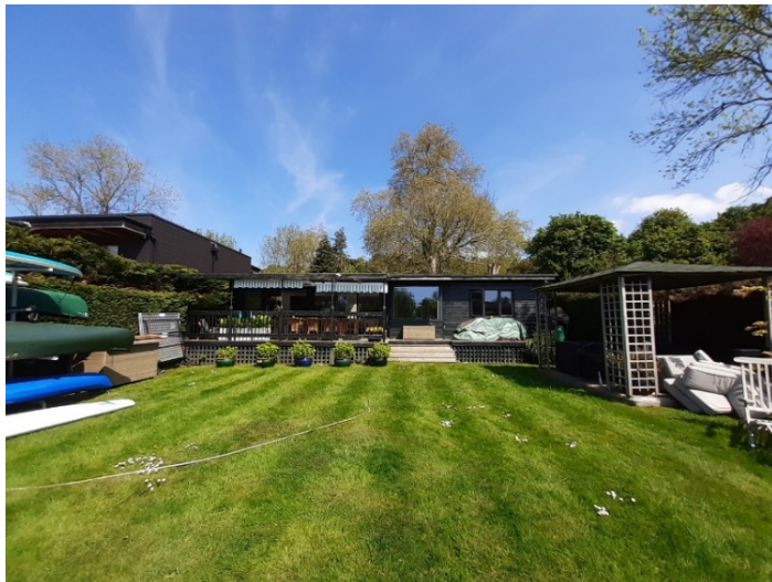
Figure 1: View of application site from the riverbank.
